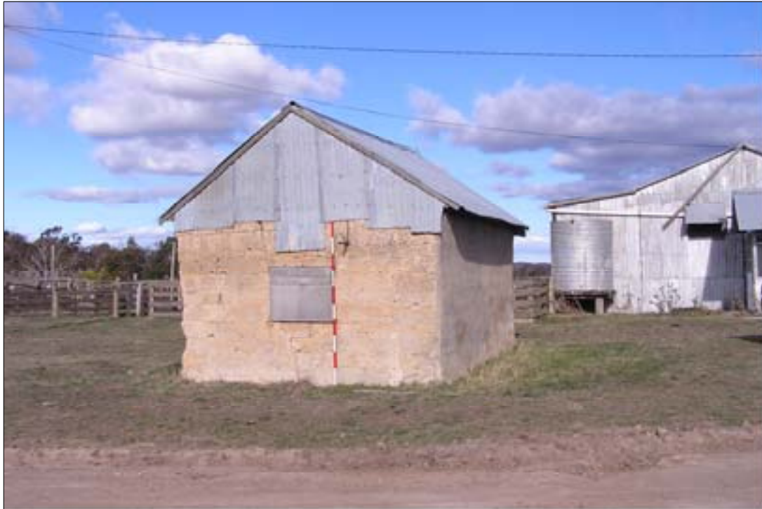
PLATE 2.23 Site MRNH5 External view of western and southern elevation of pisé building. Facing east. Shearing shed visible background right. Scale 200mm
