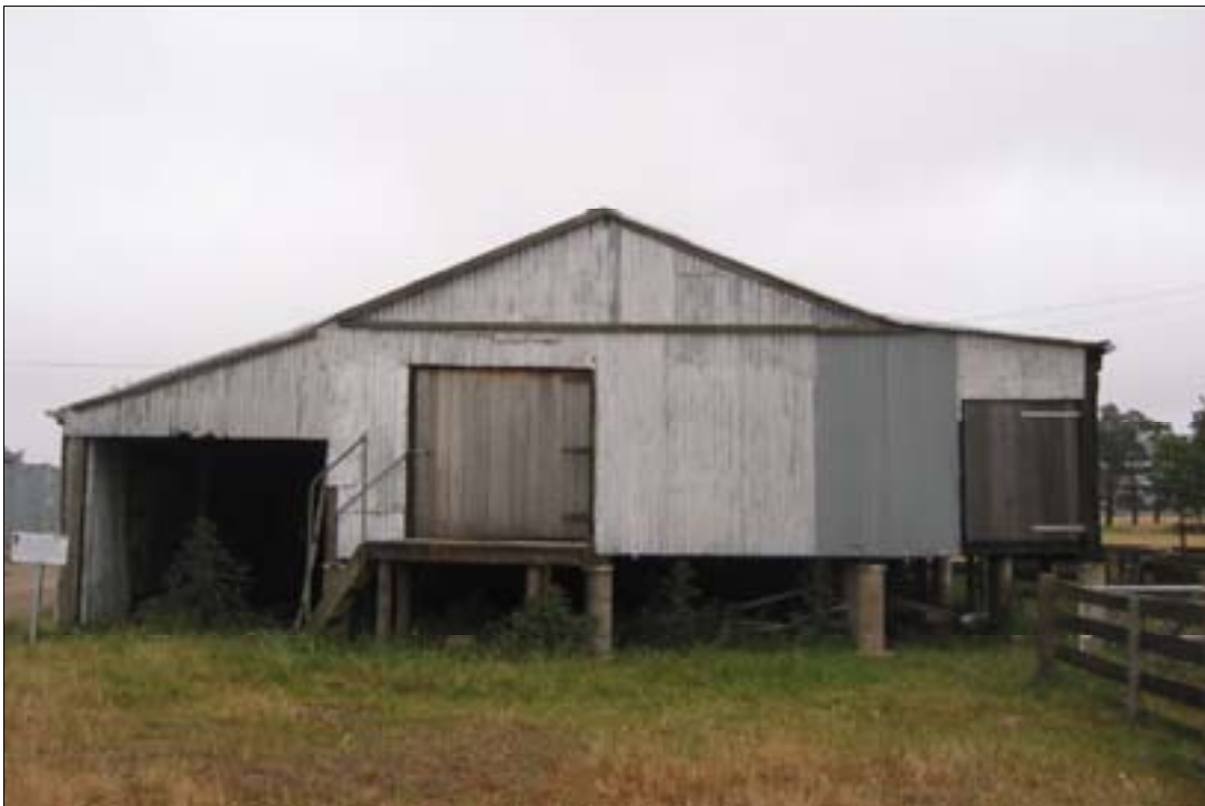
PLATE 2.12 Site MRNH5 Eastern elevation of shearing shed
