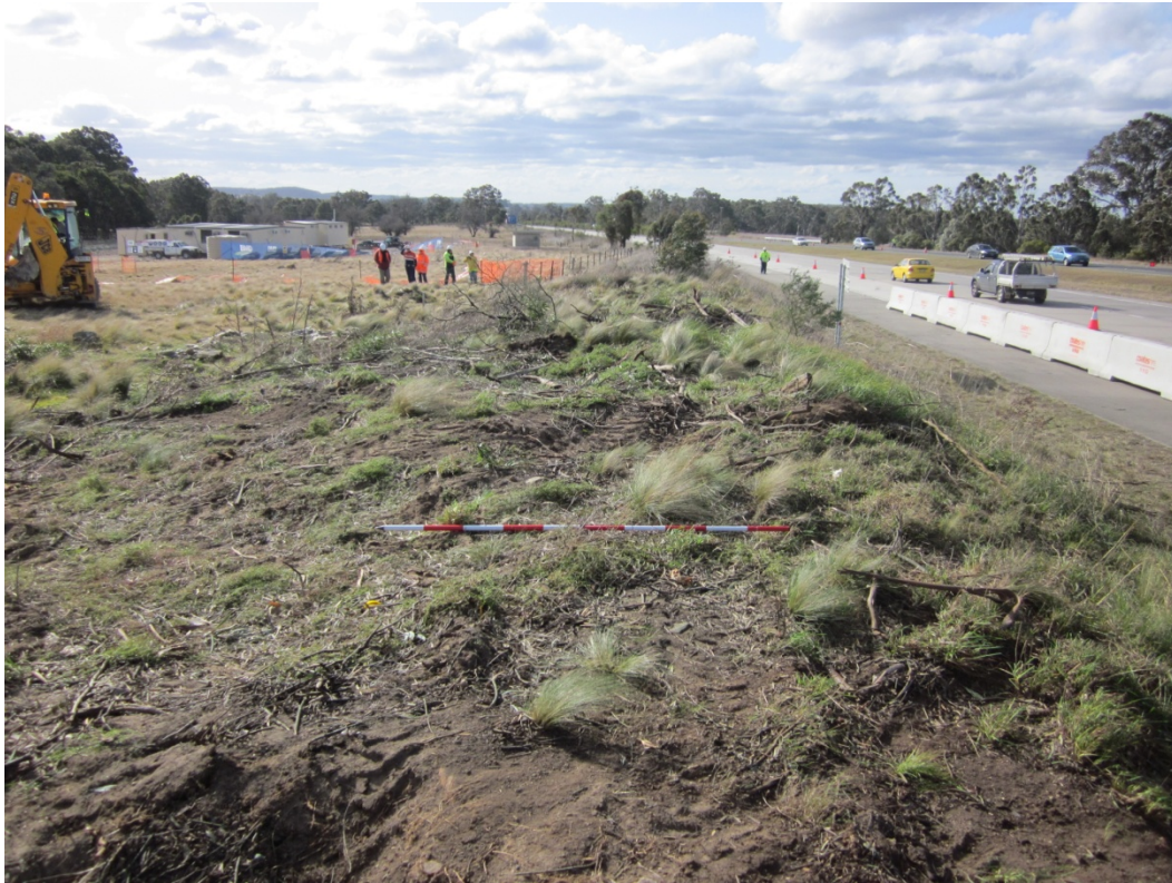
Figure 6.30. Road Reserve area following removal of trees in 2011
