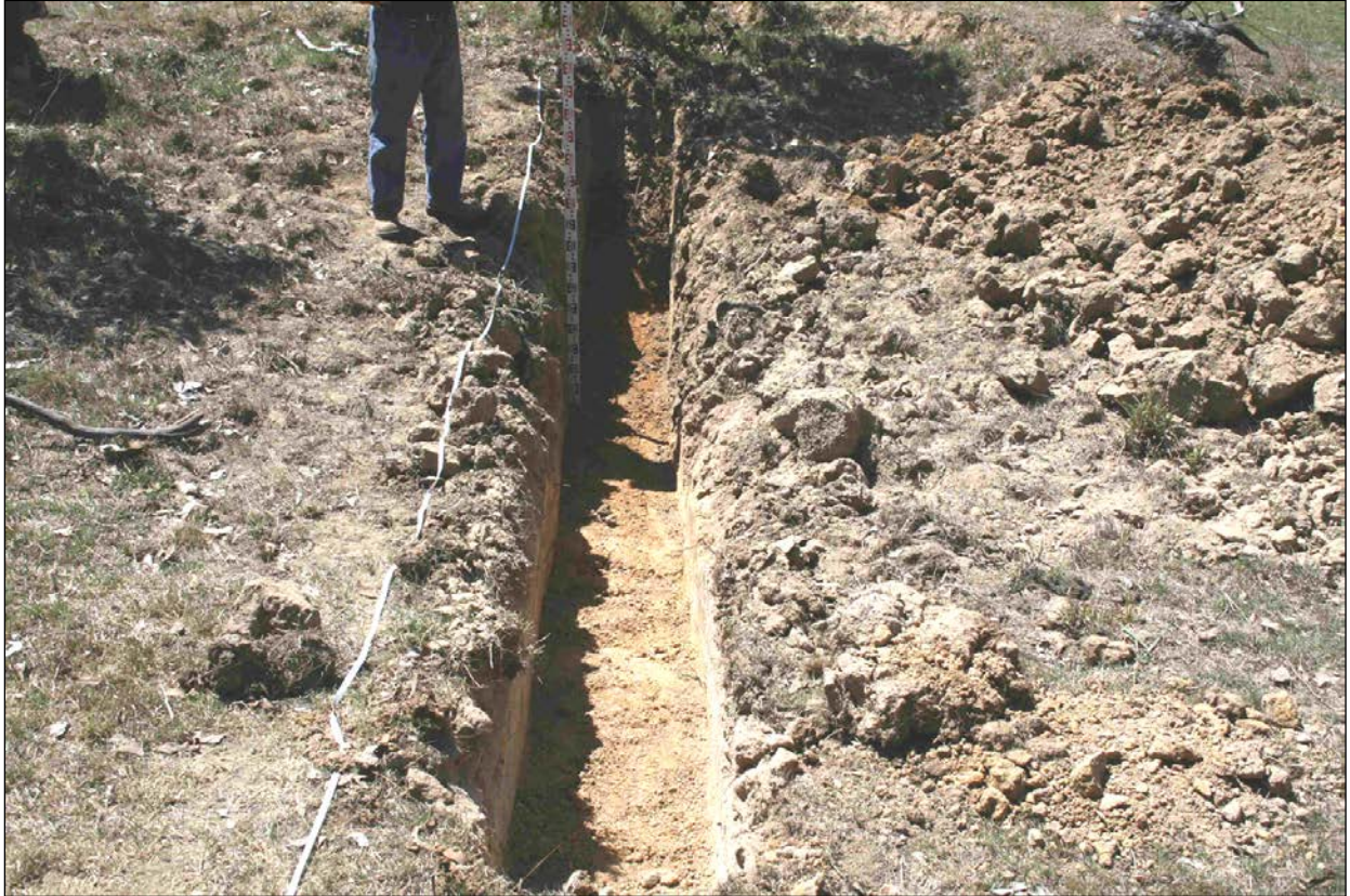
Figure 6.6 – OMF 20, facing west, showing backhoe trench.
