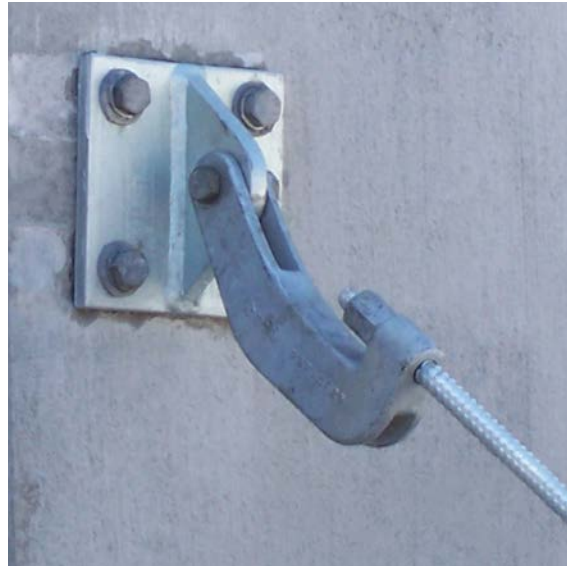
Top: Spandrel connection
