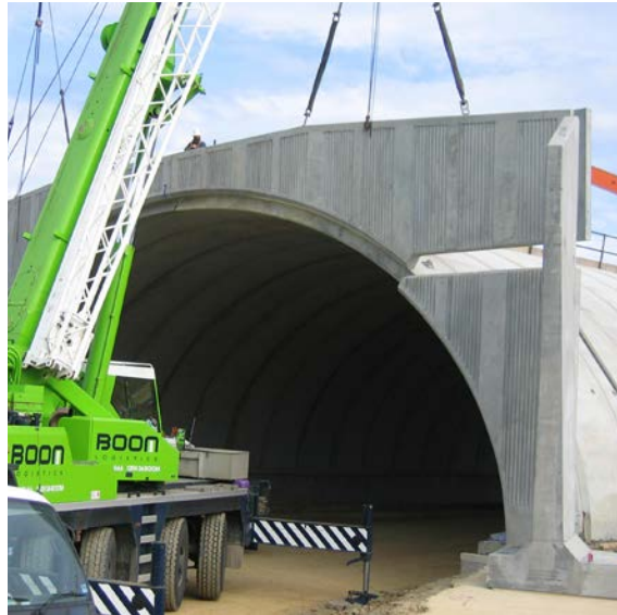
Left: Upper spandrels being joined and lowered into position
