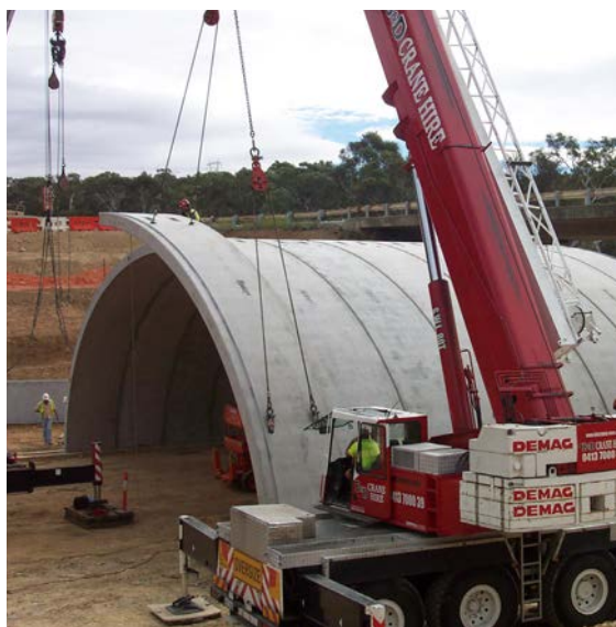
Top: Arch units being lifted into position using two cranes
