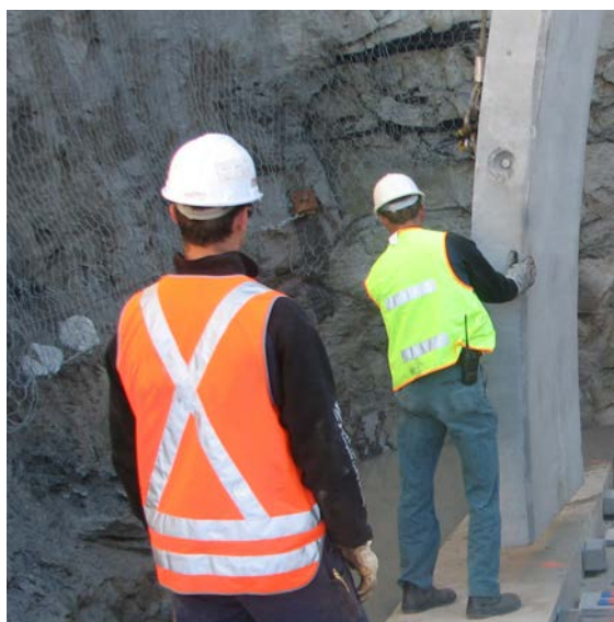
Left: Humes site representative observing installation
