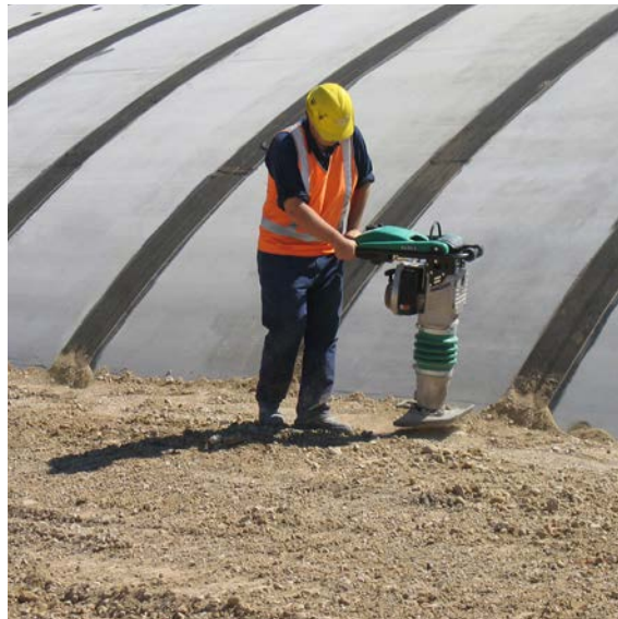
Left: Hand compaction of backfill
