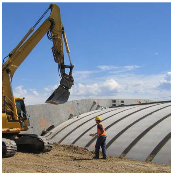
Top: Joints sealed, checking backfill
