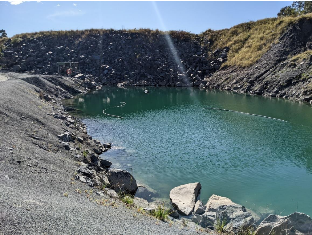
Water storage area in the main pit, able to be pumped into the primary sedimentation pond
