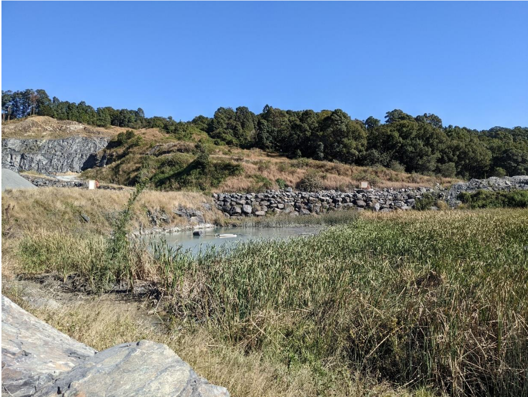
Primary sedimentation pond with visible aquatic plant growth
