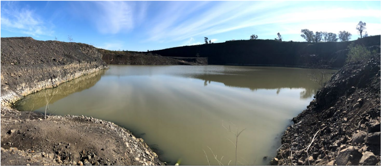
Photograph 4.1 East Pit/In Pit Dam (looking west)
