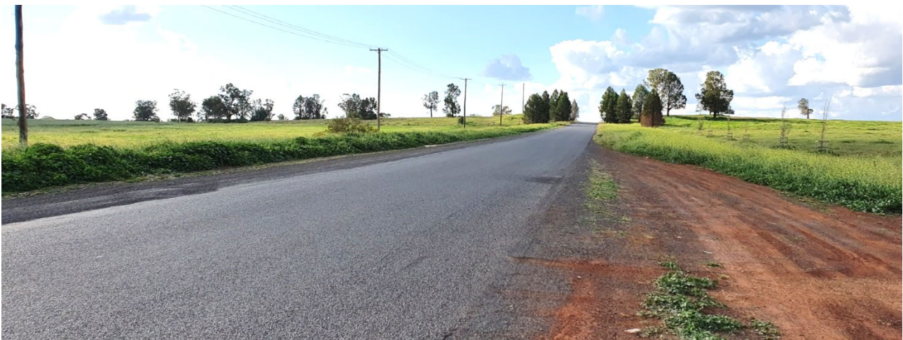
Photograph 2.2 Sheraton Road south of the schools (northbound)
