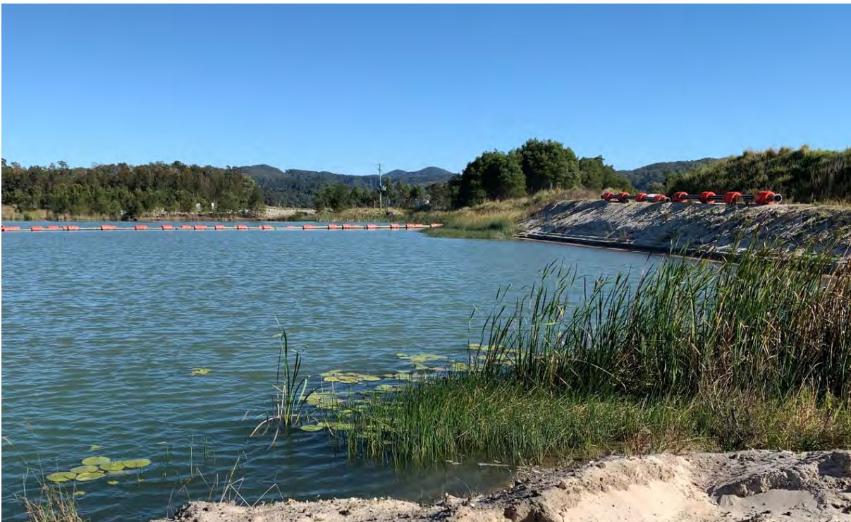
Figure 14 Fines return line Pond 1 and additional fines return line
