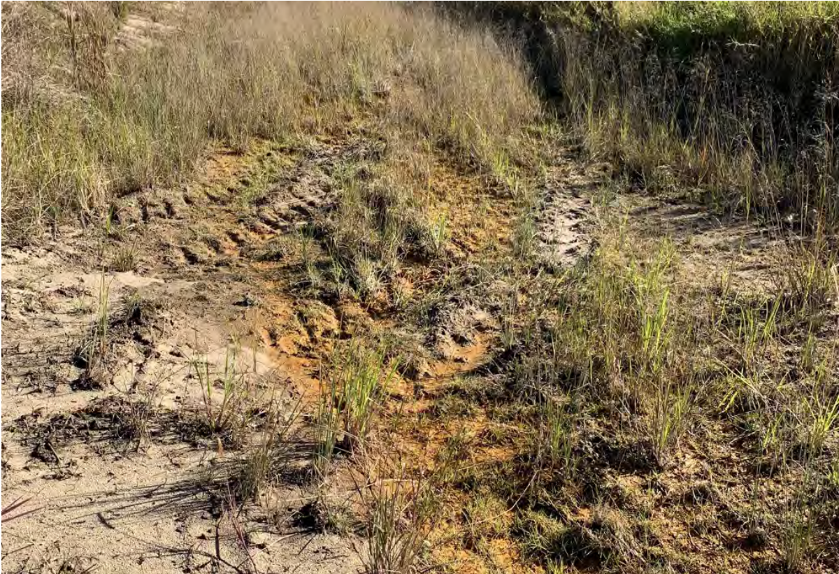
Figure 13 Sand staining from acid sulfate seepage return to Pond 2, Note: Grass growth tolerant of acidic conditions
