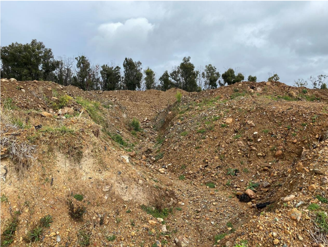
Plate 1 Potential for erosion along the outer edge of the Overburden Stockpile area.
