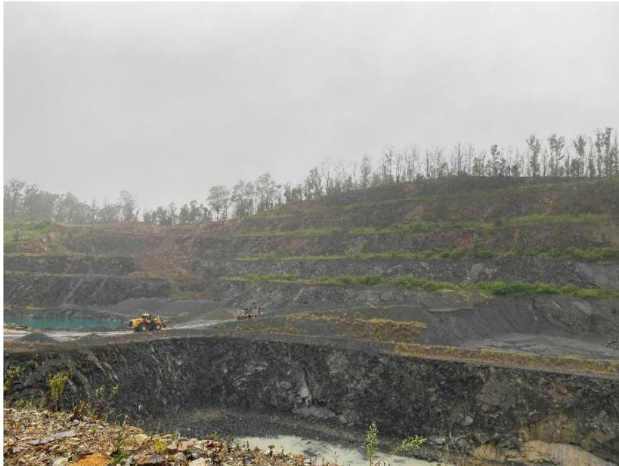
Plate 3: View of the rehabilitated benches from RL 62 looking southeast.
