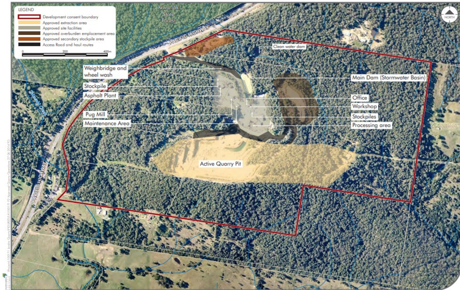
Figure 2: Jandra Quarry Operation – Source: Umwelt August 2012
