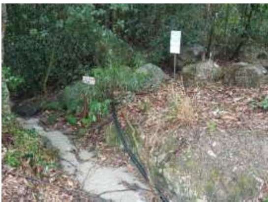
LDP at the Main Dam, with dirty water observed to be flowing past without being captured, to allow sediment to settle and water quality testing to be completed prior to re-use or discharge via the LDP
