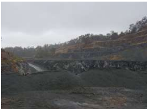
Active Pit Area at RL50, with rehabilitation of benches observed to the south and north – Facing east
