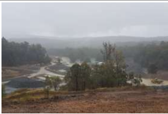
Broad overview of the site from southern boundary of the Active Quarry Pit – Facing north
