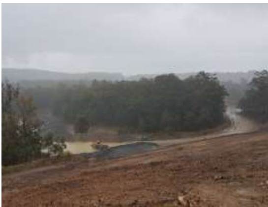
Uncleared 1.28 ha of vegetation approved for clearance – Facing generally north
