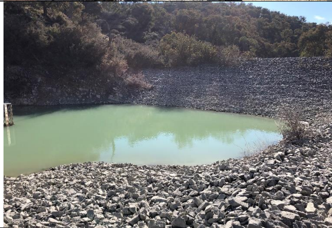
Site discharge dam for EPL Point 1
