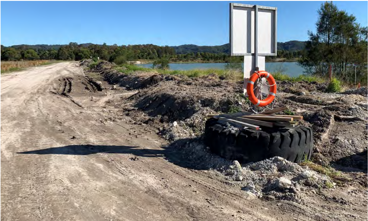
Figure 18 Soil bund along the southern edge of Pond 1
