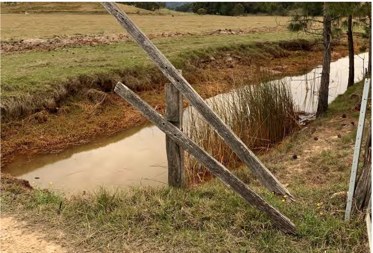
Figure 25 Typical off site drain receiving ground and surface water from pastures
