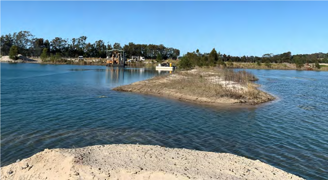
Figure 15 Opening between Ponds 1 and 2, new dredge being commissioned
