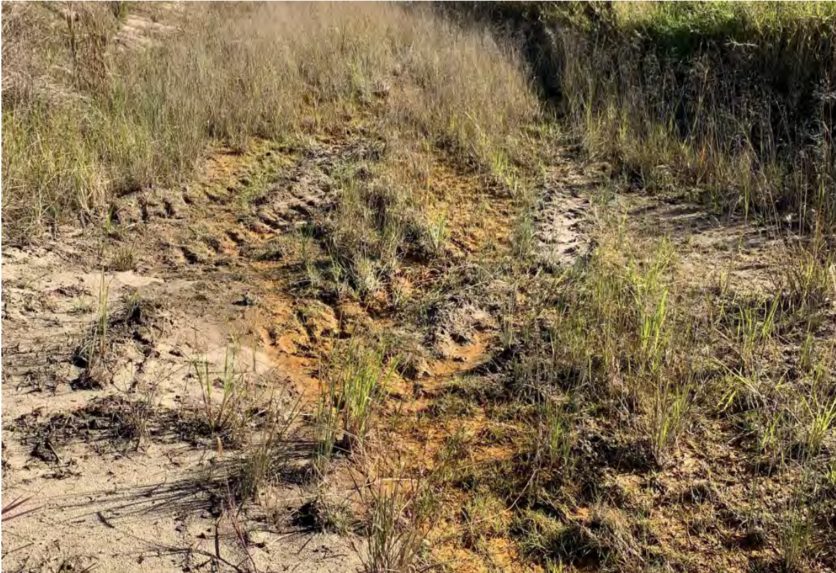
Figure 13 Sand staining from acid sulfate seepage return to Pond 2, Note: Grass growth tolerant of acidic conditions
