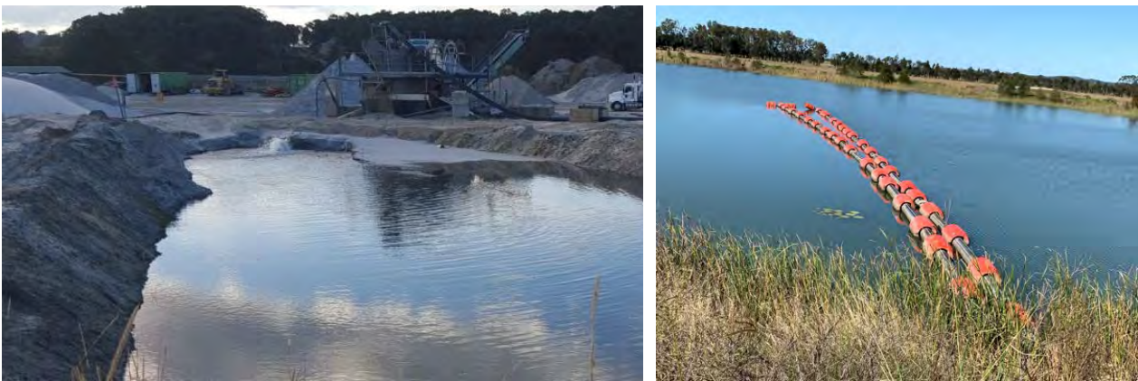
Figure 2 Fines return lagoon 2016 (left) and Pond 1 2021 (right)
