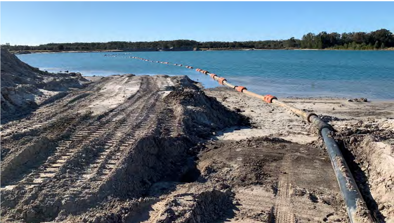
Figure 12 Dredge line from Pond 2
