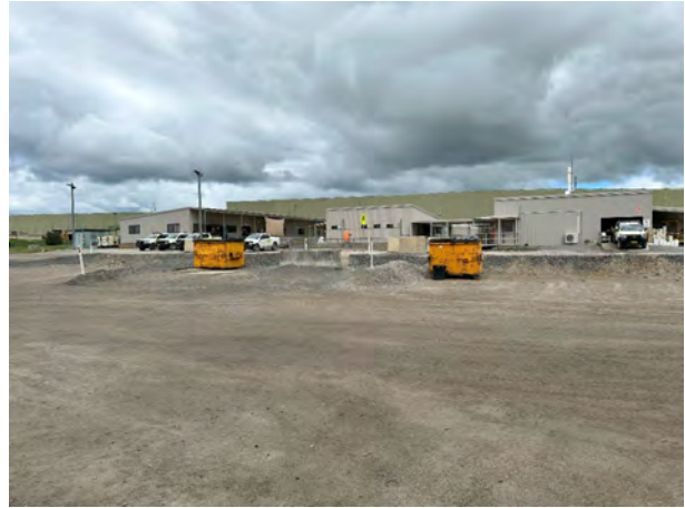
Photograph E.33 Administration area
