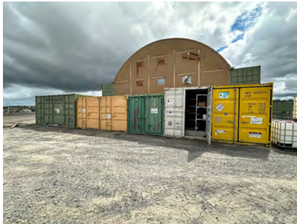
Photograph E.29 Bunded container storages for hydrocarbons
