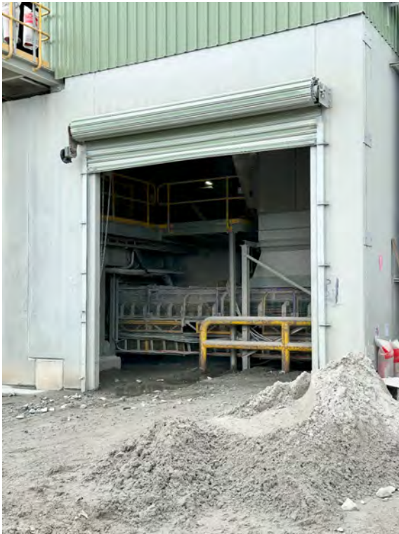
Photograph E.37 Enclosed crusher
