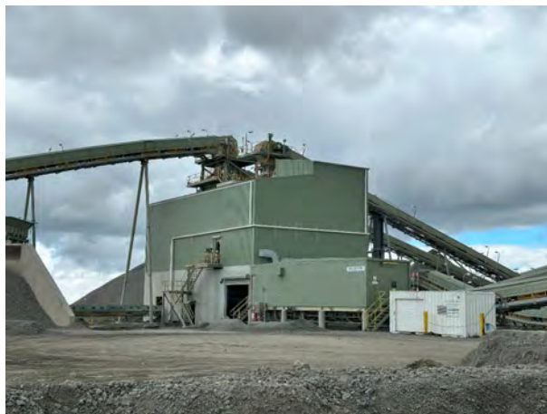
Photograph E.36 Processing plant
