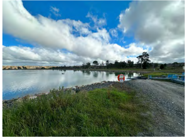
Photograph E.6 Water supply dam
