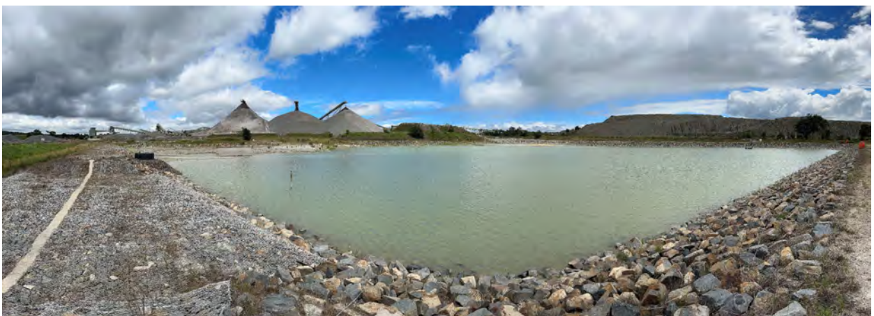
Photograph E.45 Sediment Dam E
