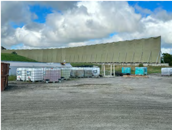
Photograph E.3 IPC located outside of bunded areas
