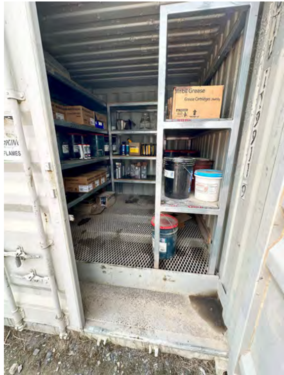
Photograph E.28 Bunded hydrocarbon storage
