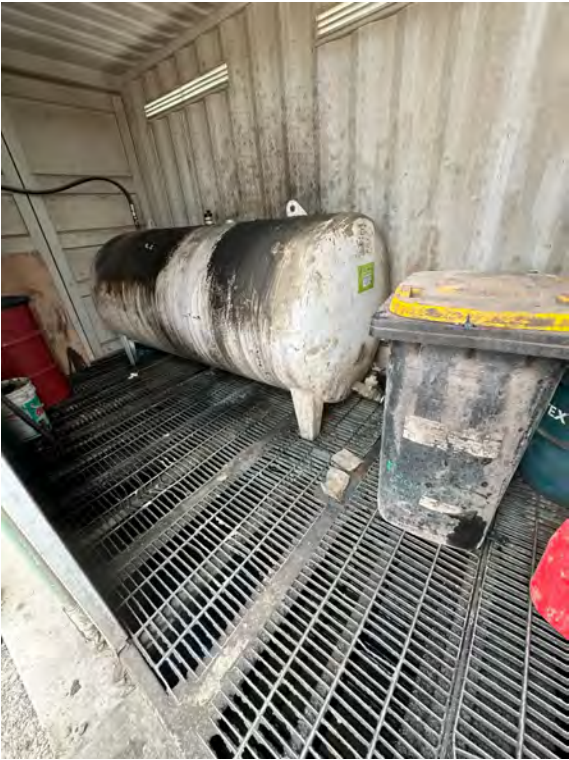
Photograph E.23 Bunded oil container
