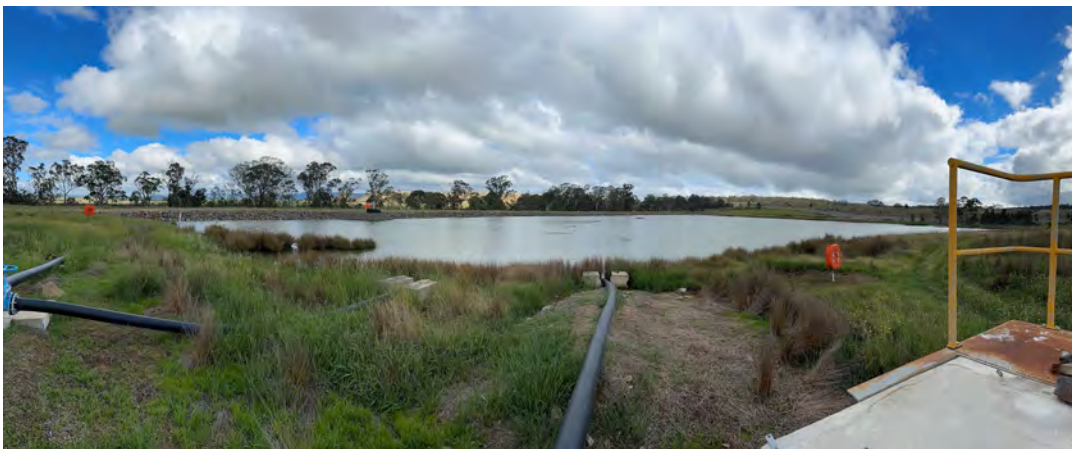
Photograph E.9 Water supply dam
