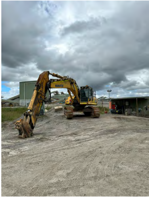
Photograph E.22 Excavator
