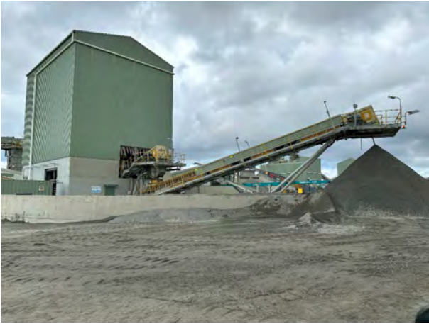
Photograph E.34 Processing plant and stacker
