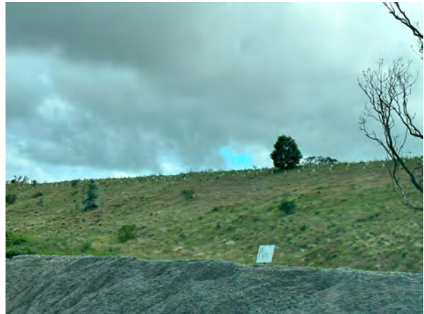
Photograph E.8 Amenity bund
