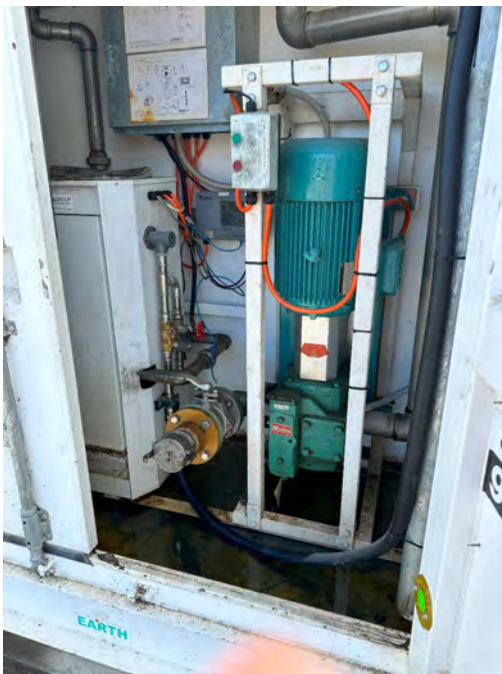
Photograph E.48 Internally banded area of truck refuelling station
