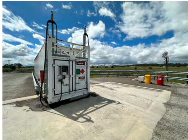
Photograph E.49 Road vehicle refuelling station
