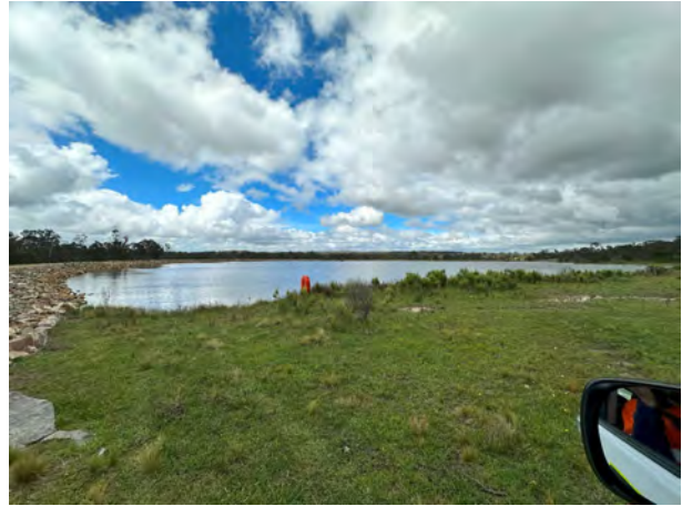
Photograph E.15 Water supply dam
