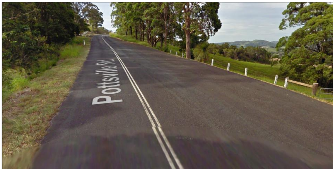
Figure 6-2 Pottsville Road in proximity to the site access intersection
