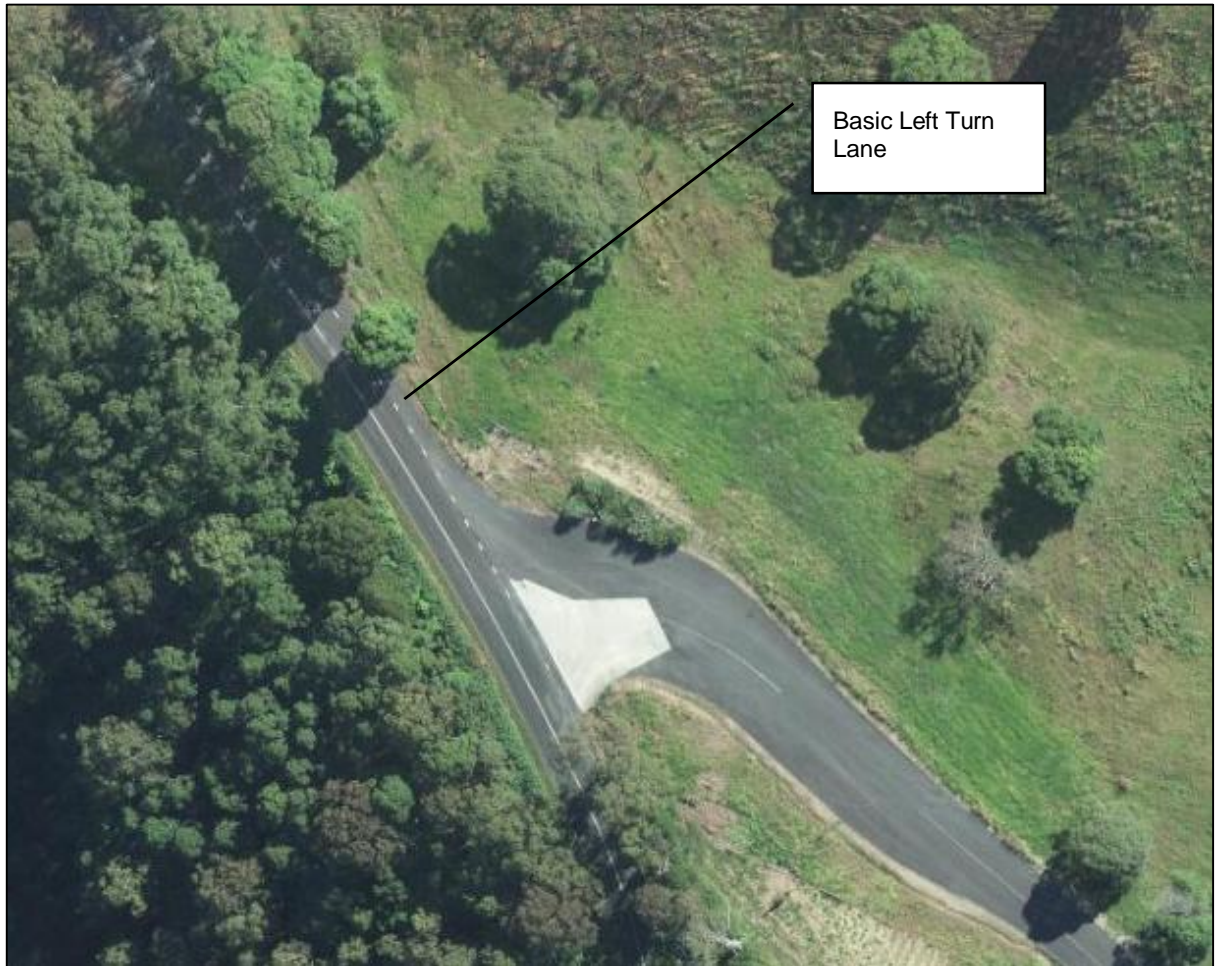
Figure 4-4 Quarry access road intersection
