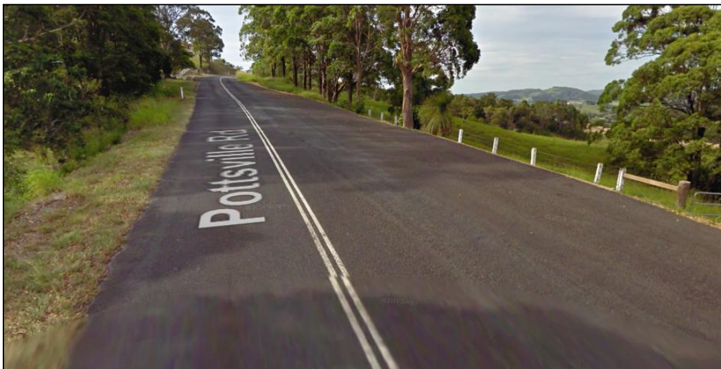
Figure 3-2 Pottsville Road in proximity to the site access intersection
