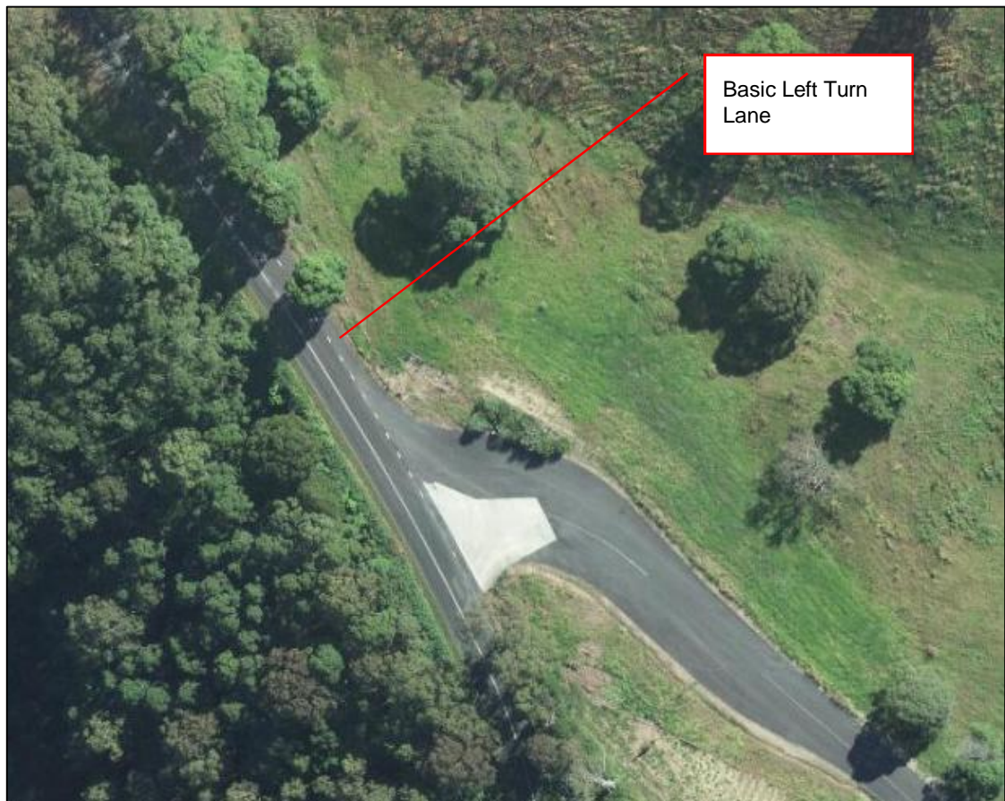
Figure 6-10 Quarry access road intersection
