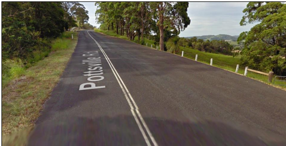
Figure 3-1 Pottsville Road in proximity to the site access intersection
