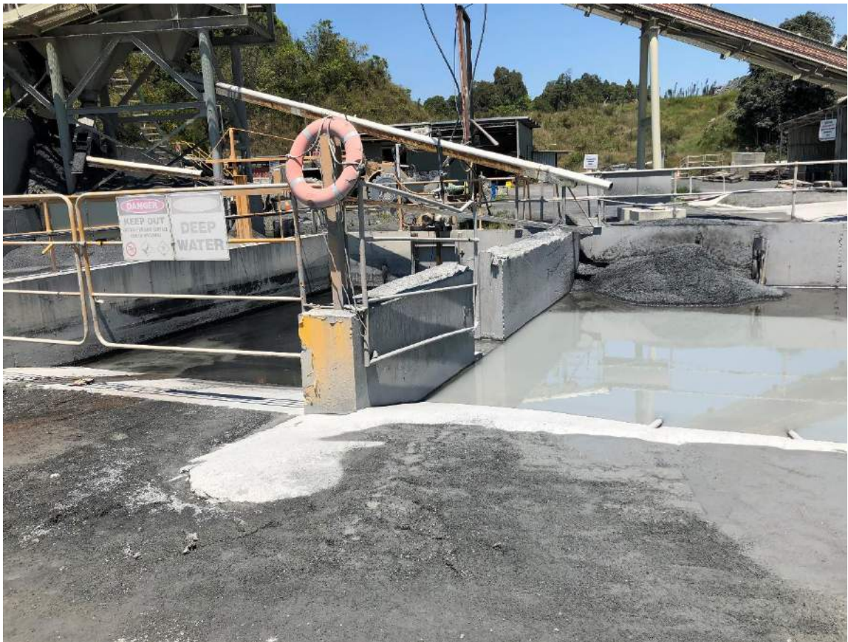
Photograph 10: Wedge pits adjacent to main processing facilities and workshop
