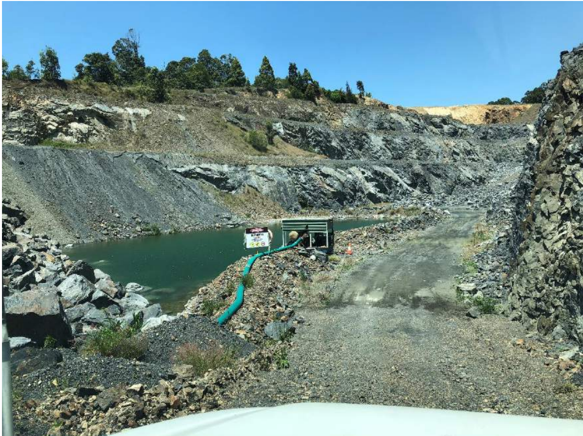
Photograph 1: Pit Dam – view to south with pump and rising main shown in foreground
