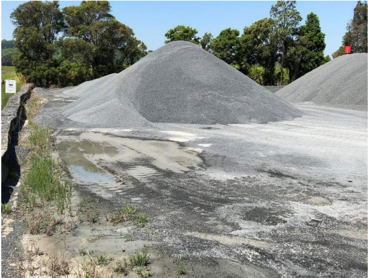
Photograph 15: Main stockpile area showing ponded runoff and concrete block bunding located along northern site boundary
