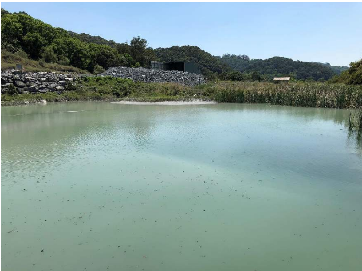
Photograph 2: Main Dam – view to north across dam
