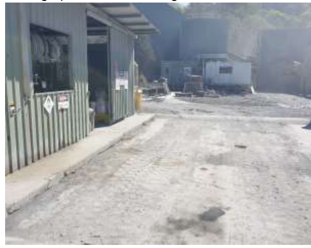
Photograph 8: Bunded refuelling area
