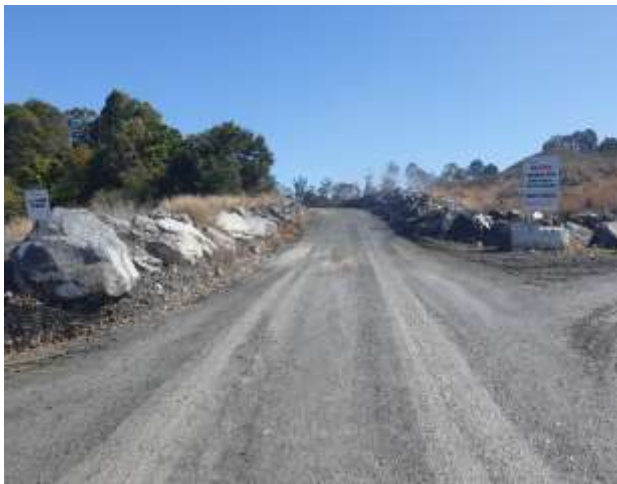
Photograph 1: A haul road with the automatic sprinklers on to control dust
