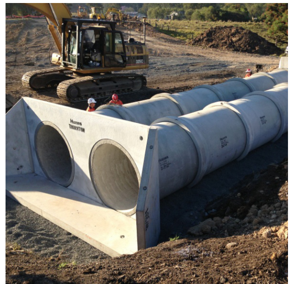
Concrete pipes and headwall structure
