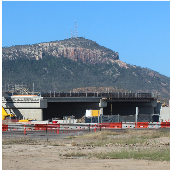
Top: Prestressed deck units – Bruce Hwy upgrade V2C
