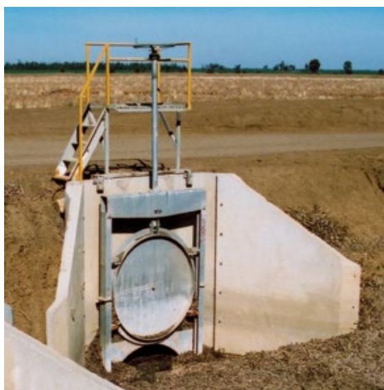
Left: Irrigation headwall with control gate
