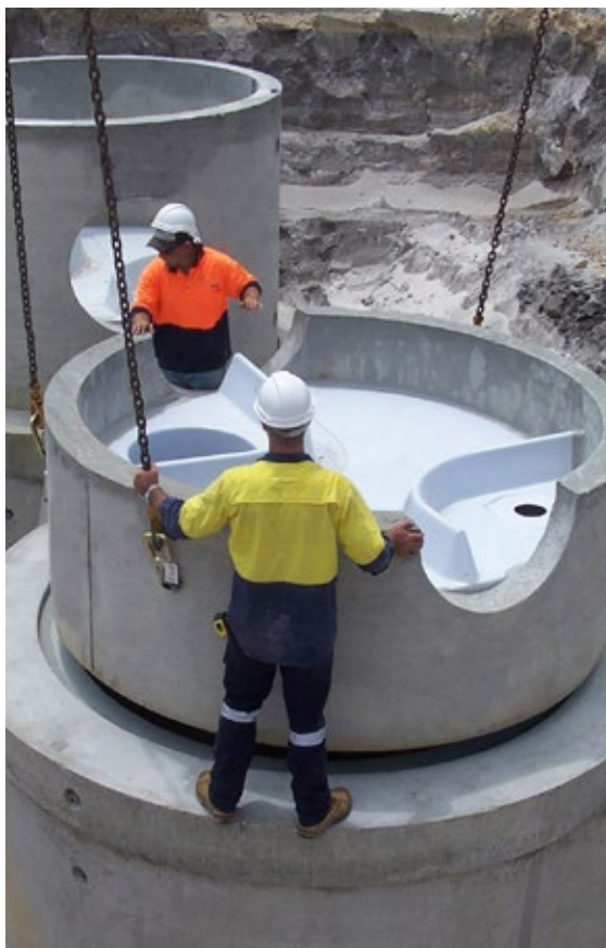
Right: HumeCeptor® system being assembled on site
