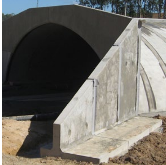
Left: Heavy type wing walls on a precast arch structure
