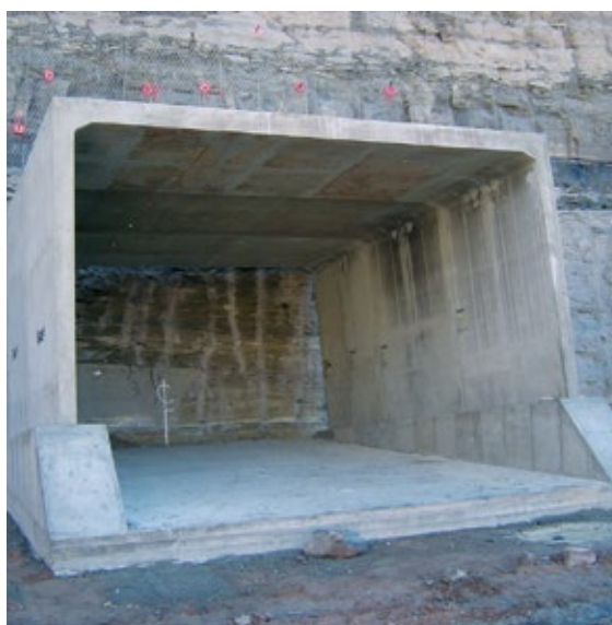
Left: 3-pin arch reclaim tunnel
