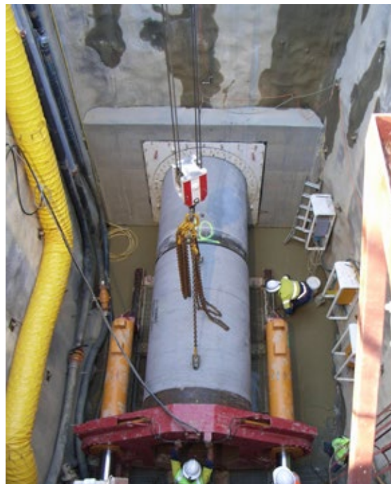
Left: J series jacking pipe installation
