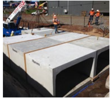
Box culverts - small 16
