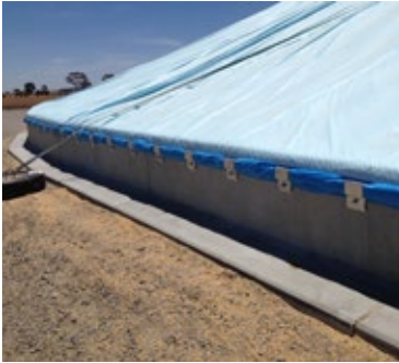
Grain bunker modules
