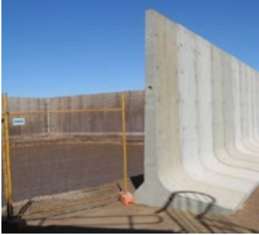
Land T walls
