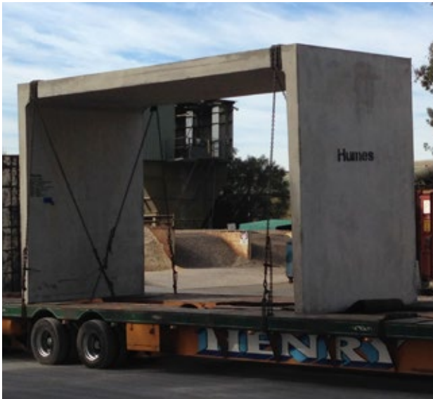
Large box culverts
