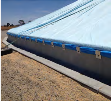
Grain bunker modules
