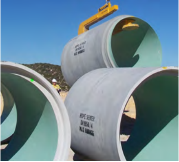
SRC pipes with corrosion protection 25
