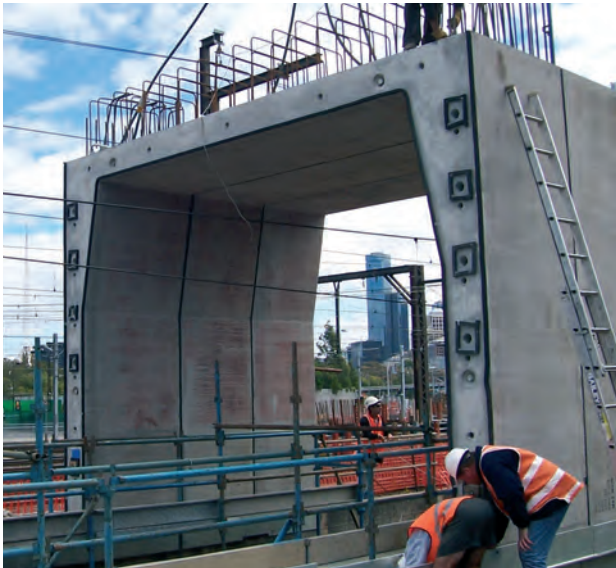
Box culverts with post-tensioning ducts
