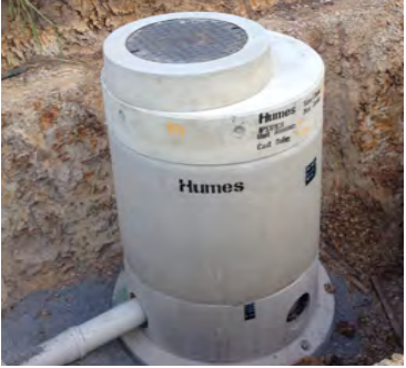
Access chambers/Manholes 27
