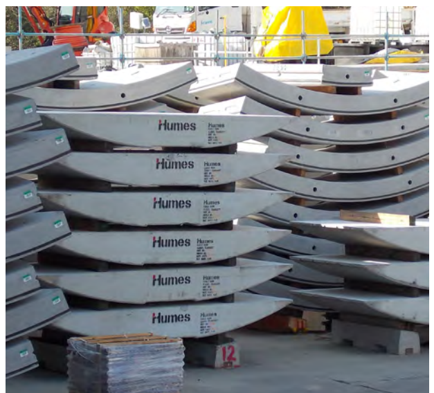
Tunnel invert units
