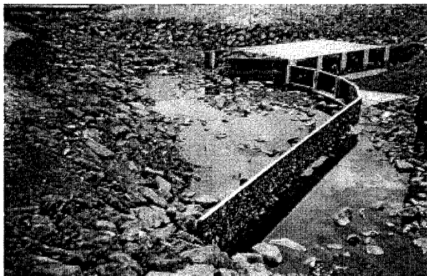
Plate 2.16 Contra-shear diversion weir with net bagging system downstream of Preston Main Drain, Melbourne (Author's photograph, 2003).
