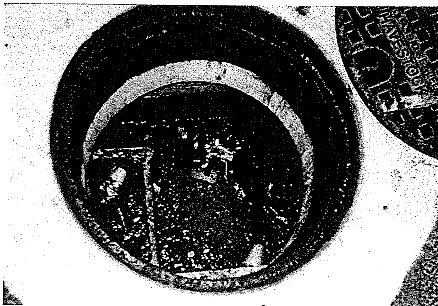
Plate 5.2 Litter and oil on the surface of the holding chamber of the Toombah Street ILLS prototype (Authors Photograph, November 1997)
