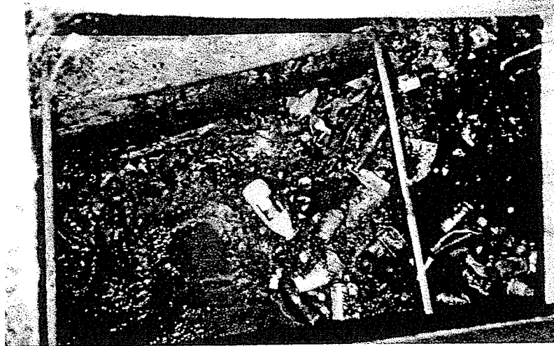
Plate 5.19 O'Grady Street prototype. Boom separator chamber clogged with gross pollutants following a lack of cleaning (Authors photograph, May 2003).
