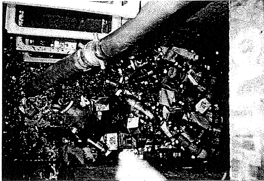
Plate 5.15 Youth Road ILLS prototype holding chamber showing litter on surface and vacuum street sweeper truck hose retrieving litter (Authors photograph, 30 September 1998).
