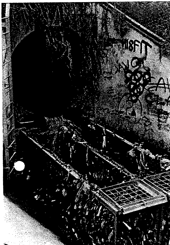
Plate 2.12 Litter cage at drainage outlet (Author's photograph, 1998).
