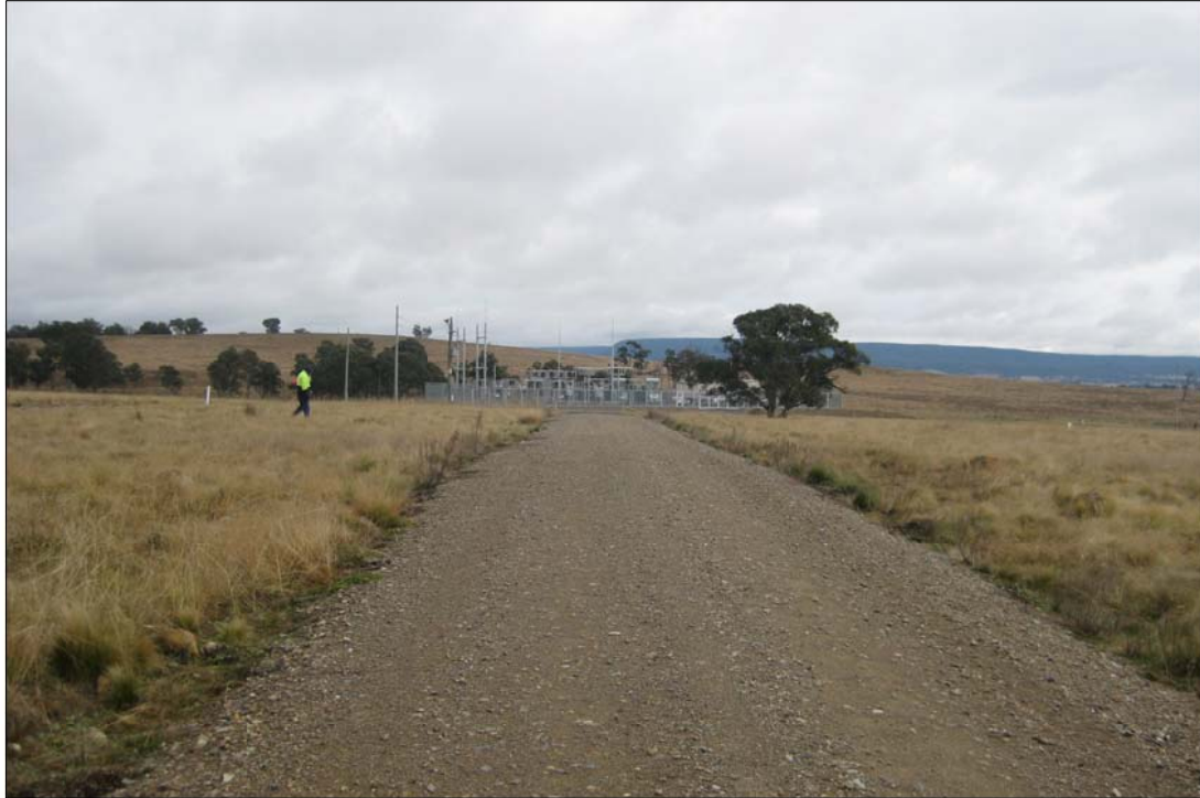
PLATE 22 Part PAD2 Area facing west towards North Marulan Zone Substation and MRN54 site
