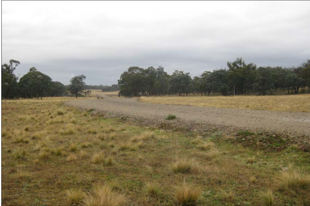
PLATE 1 MRN15 - access track constructed on geotextile facing E
