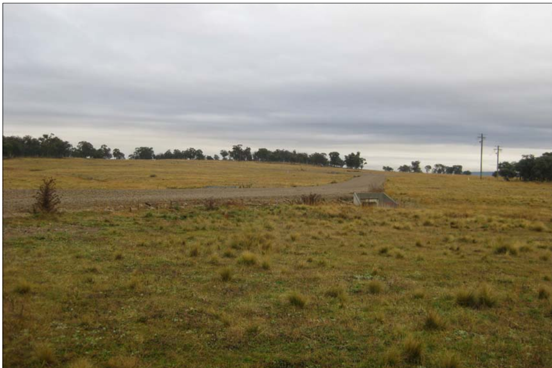
PLATE 2 Transect 1 Joarimin Creek crossing to north of MRN15. Showing culvert and road constructed on geotextile
