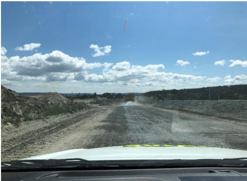
Figure 9: Dust suppression occurring via water cart on aggregate road
