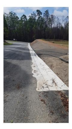
Photo 2: Kerbside drain and gutter installed at the main Jandra Quarry driveway
