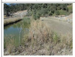
Settling ponds (one being active and the other dewatering at any one time)
