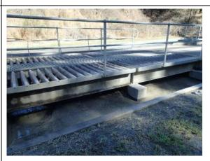
Shaker system at the site exit, which trucks pass over following the wheel wash. Excess water is drained and cycled through the wheel wash, while material is collected for disposal
