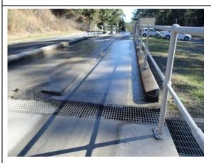
Wheel wash system at the site exit, with water cycled through via a pump before draining to the Main Dam for reuse.
