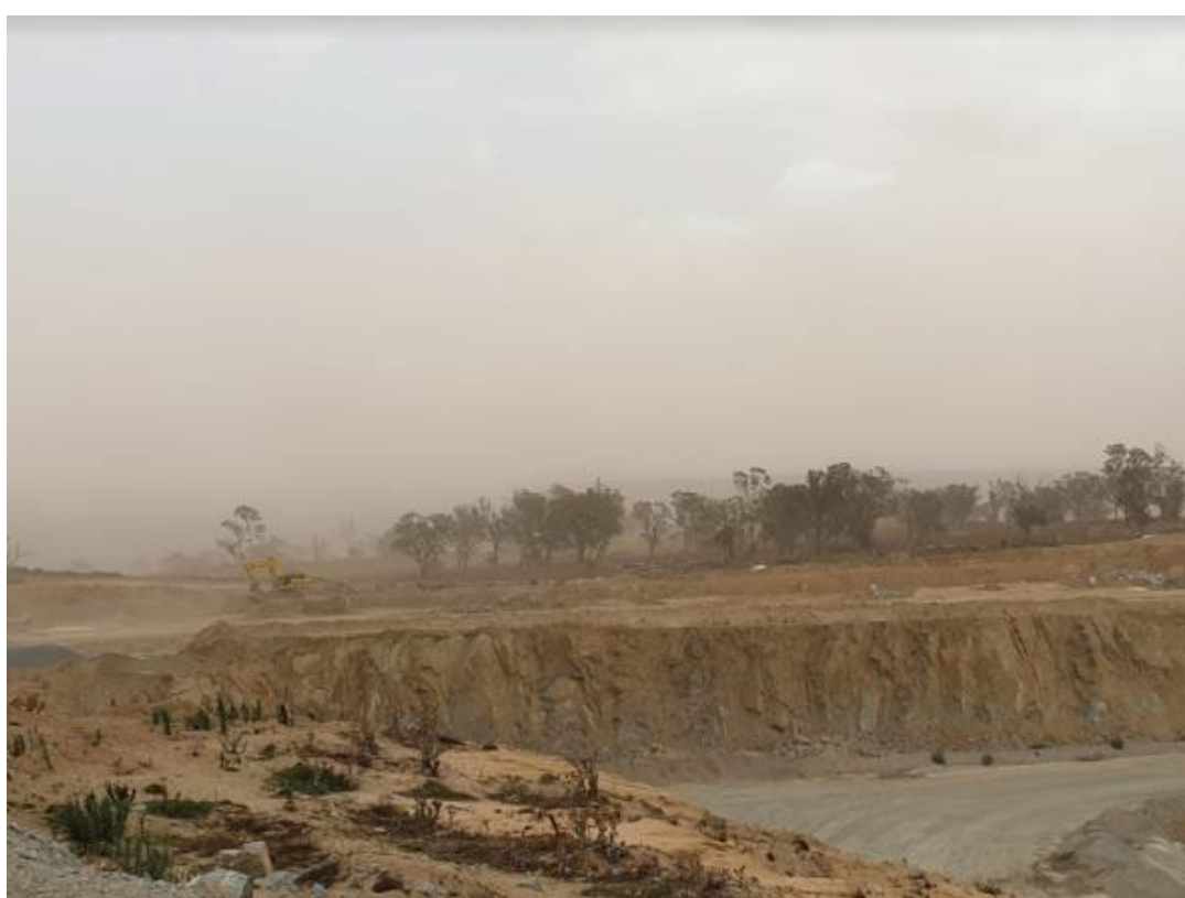
Figure 6: Photograph taken on site of weather conditions on 23/01/2020.
