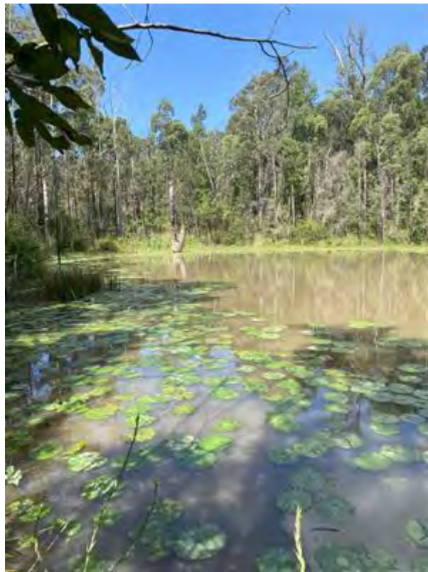
Plate 2 Dam below rehabilitated area.
