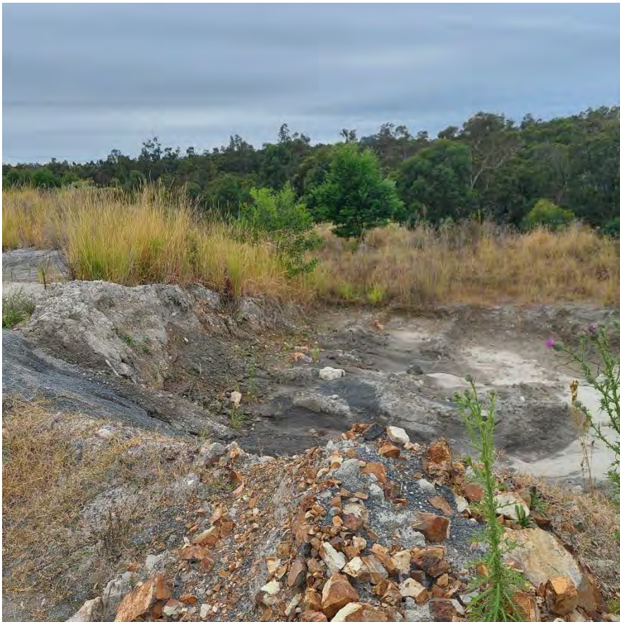
Plate 10 Erosion control / point in Overburden Stockpile Area.
