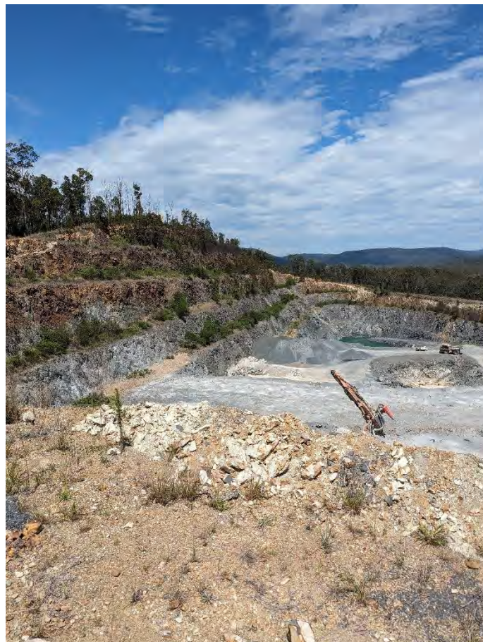
Plate 4 Rehabilitated benches along the eastern side of the AP area.
