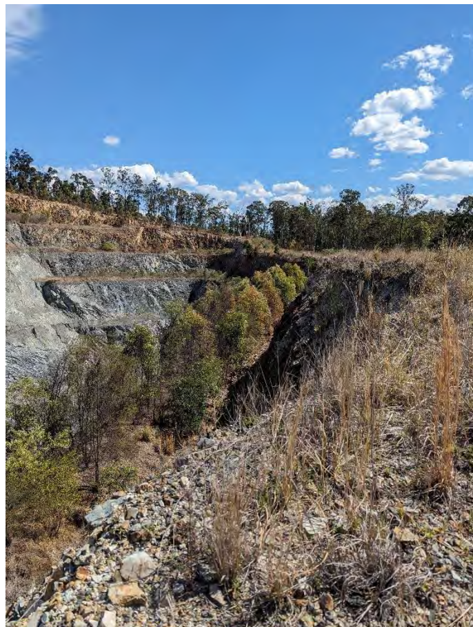
Plate 6 Under-cut from erosion along the high-wall of the western AP area.
