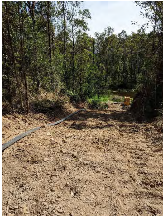
Plate 10 Access track to lower Dam Location.
