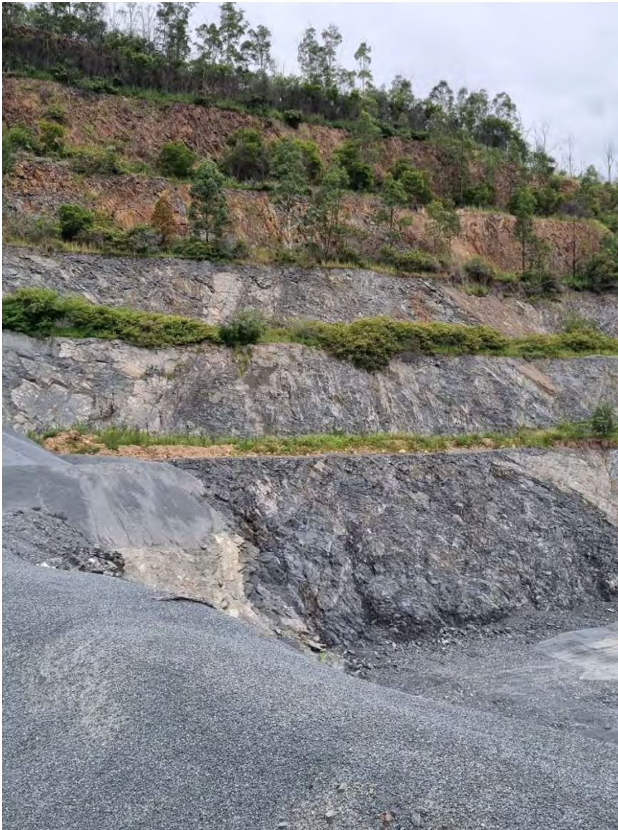
Photo 1: Active Rehabilitation of benches at Jandra Quarry (2023)
