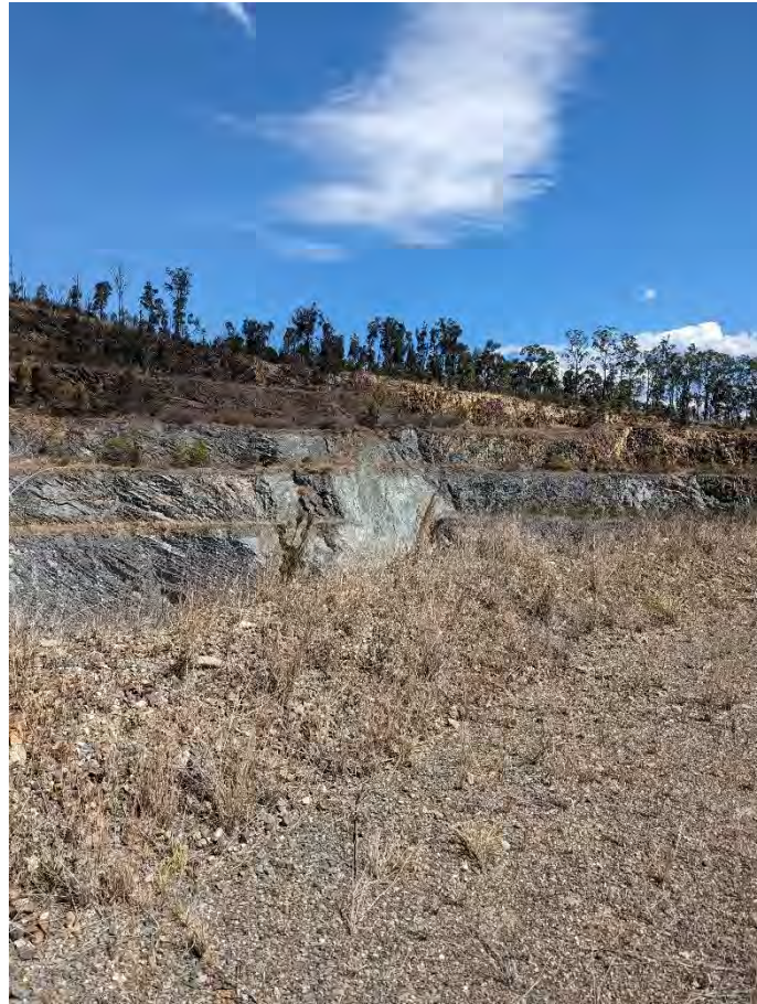
Plate 5 Rehabilitated benches along the eastern side of the AP area.
