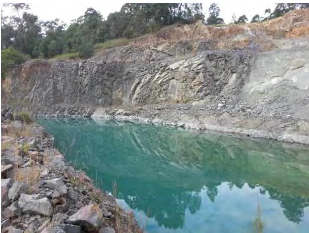
Plate 4: The pit dam. A sump created in the floor of the quarry to capture sediment laden stormwater runoff from the quarry pit.
