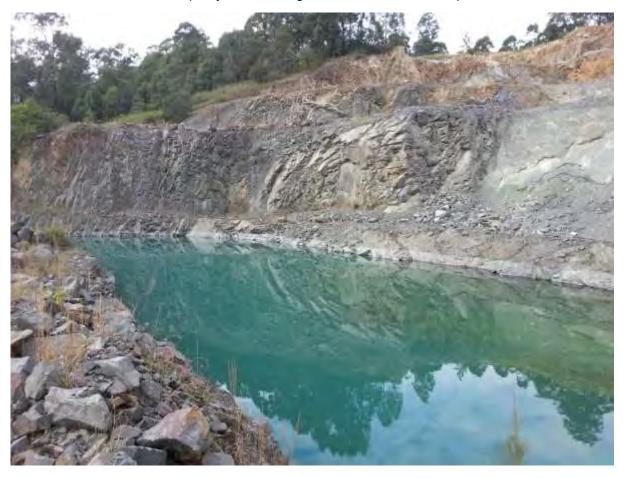
Plate 4: The pit dam. A sump created in the floor of the quarry to capture sediment laden stormwater runoff from the quarry pit.
