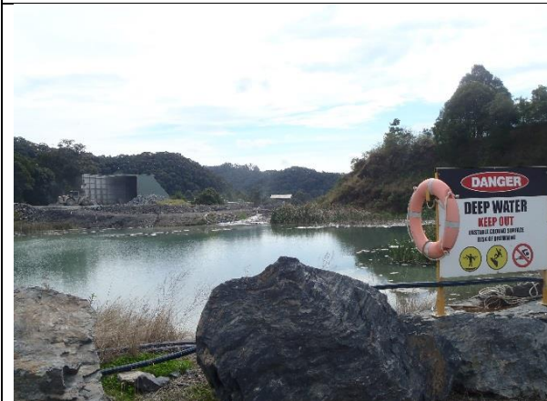
The Main Dam, with a total volume of approximately 11.5 ML.
