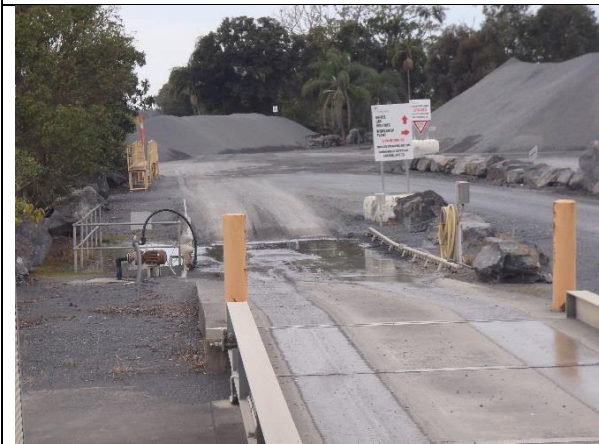
Wheel wash system at the site exit, with a truck wash area and product stockpiles in the background. Water is recycled back to the Main Dam?
