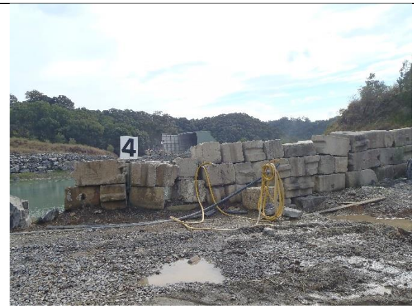
Truck wash area between the Main Dam and Haul Road.
