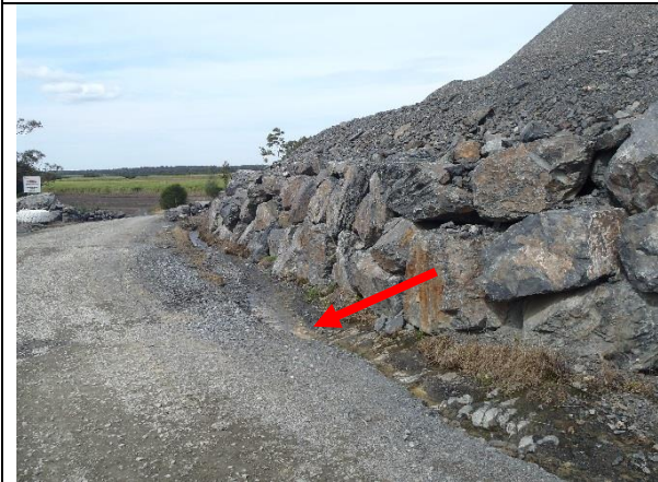
The Main Dam discharge point, out of dam.
