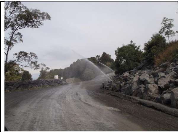
Sprinklers in operation on the haul road to manage dust generation.
