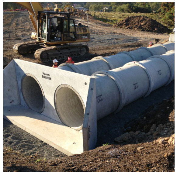
Concrete pipes and headwall structure
