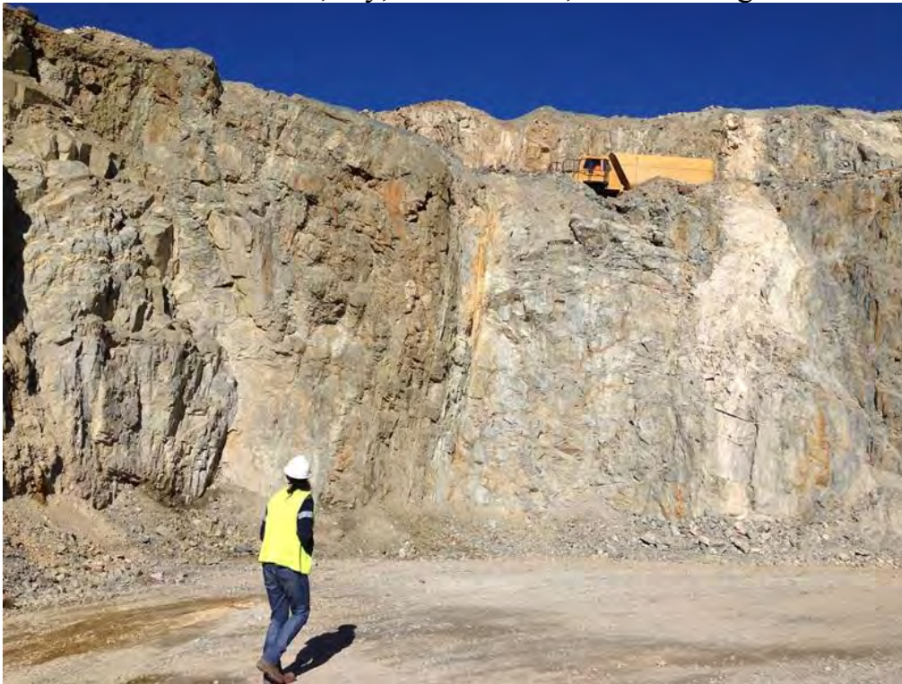
c Bench 3 rock face, dry, in Dacite Pit, southern edge
