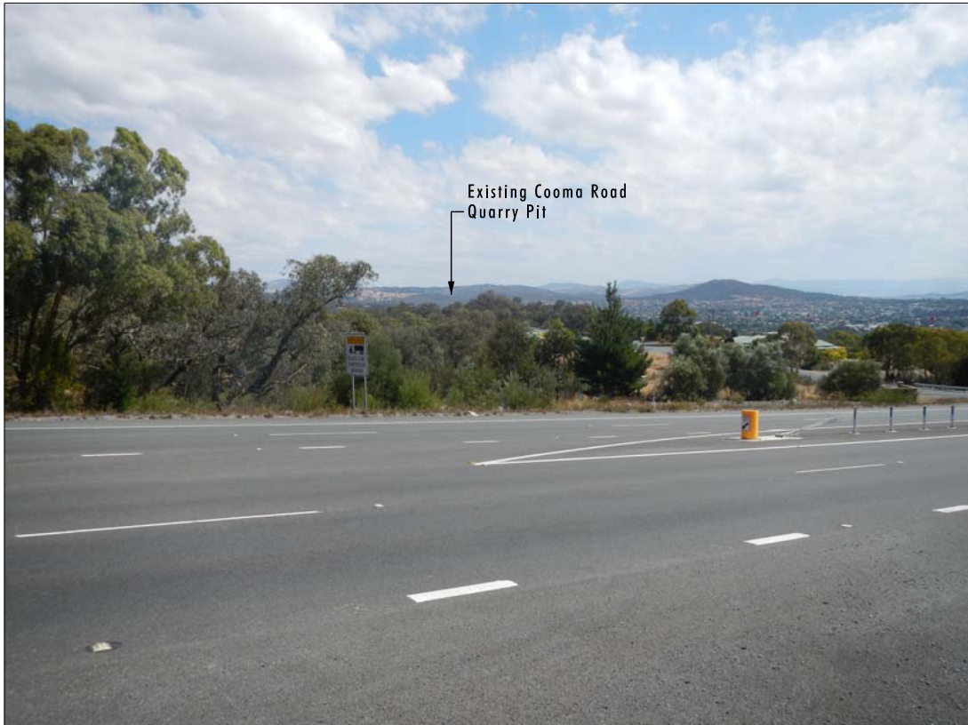
PLATE 2.1 View of Cooma Road Quarry - Intersection of Kings Highway and Hills Lane
