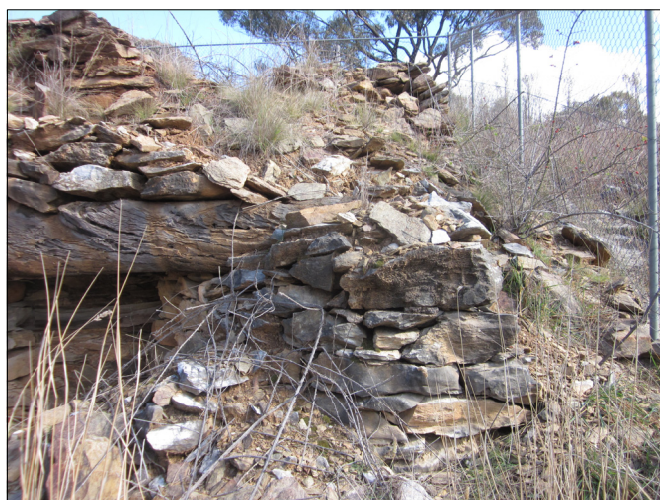
PLATE 3.5 May 2012 photograph of kiln structure, view to west
