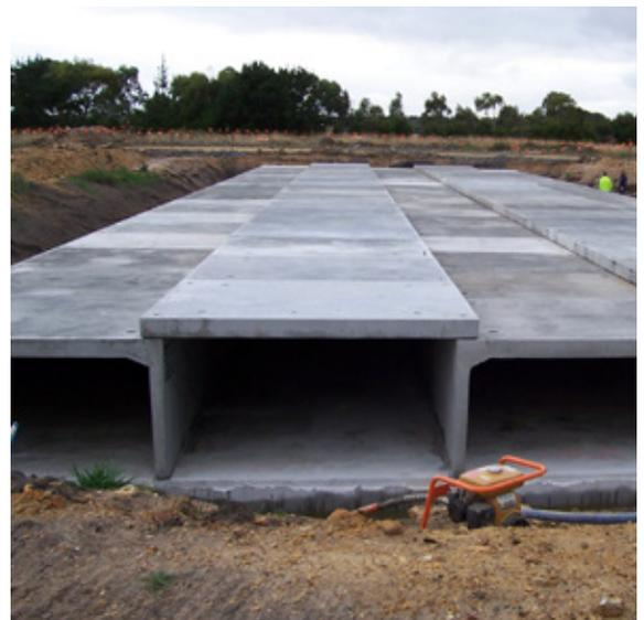
Figure 2 – General layout of a multi-cell installation using Link Slab® units
