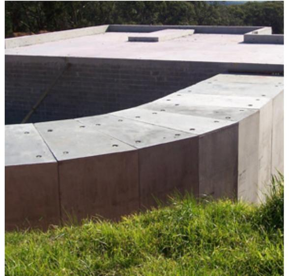
**Figure 3 – Typical two cell box culvert layout of skewed angles up to  $25^\circ$**
