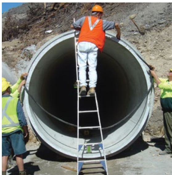
Left: Large diameter Rubber Ring Joint (in-wall) pipe installation
