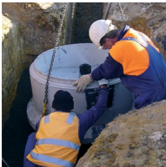
Top: Access chamber base
