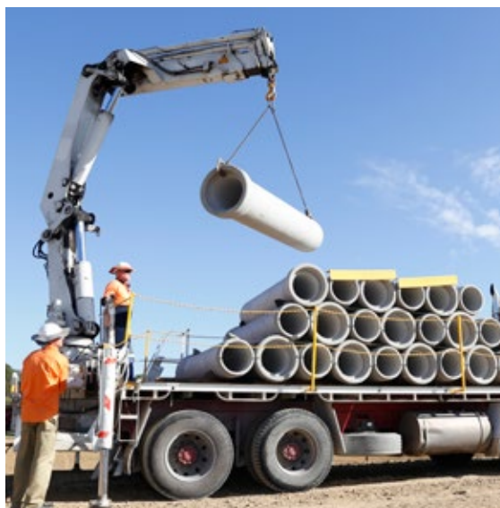
Top: Concrete pipe delivery
