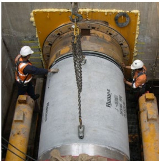
Top: Launch shaft showing exit opening and jacking station
