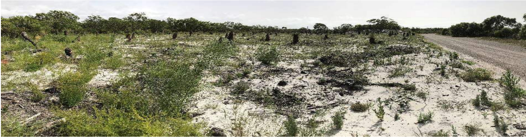
Plate 32: Block Q3 south (looking east along haul road) January 2019
