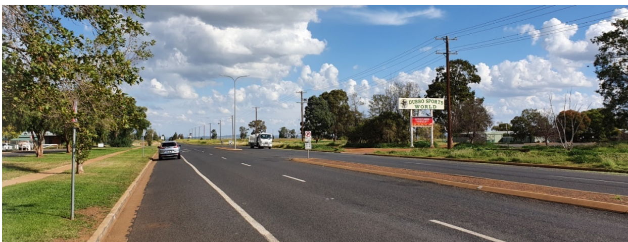
Photograph 6.2 Sheraton Road (southbound carriageway)
