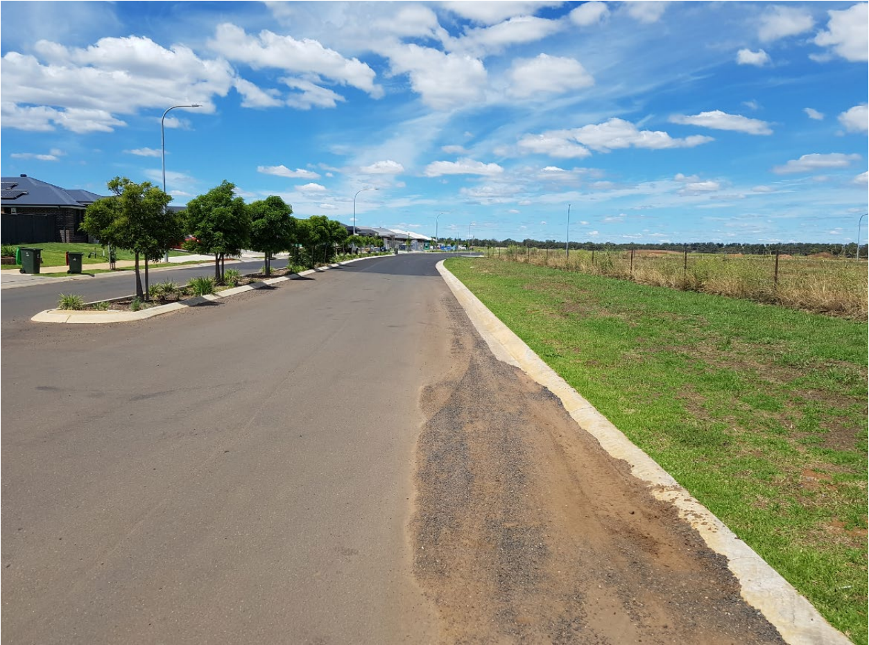
Photograph 6.4 View east from R18 Argyle Avenue, Southlakes Estate
