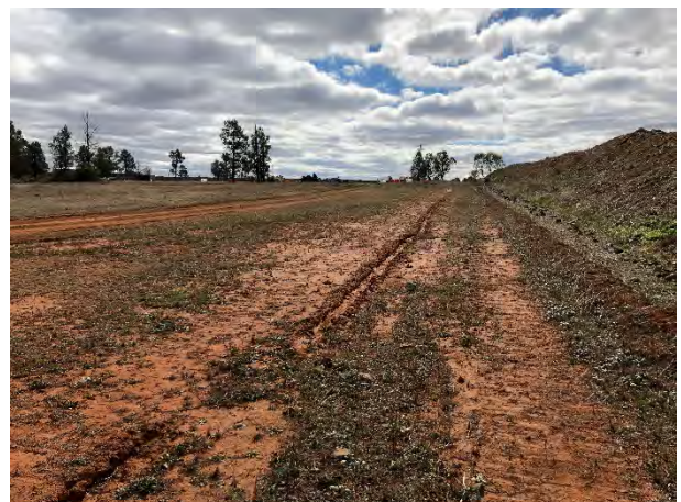
Plate 5.12 Eastern SU2. Graded disturbance. View north
