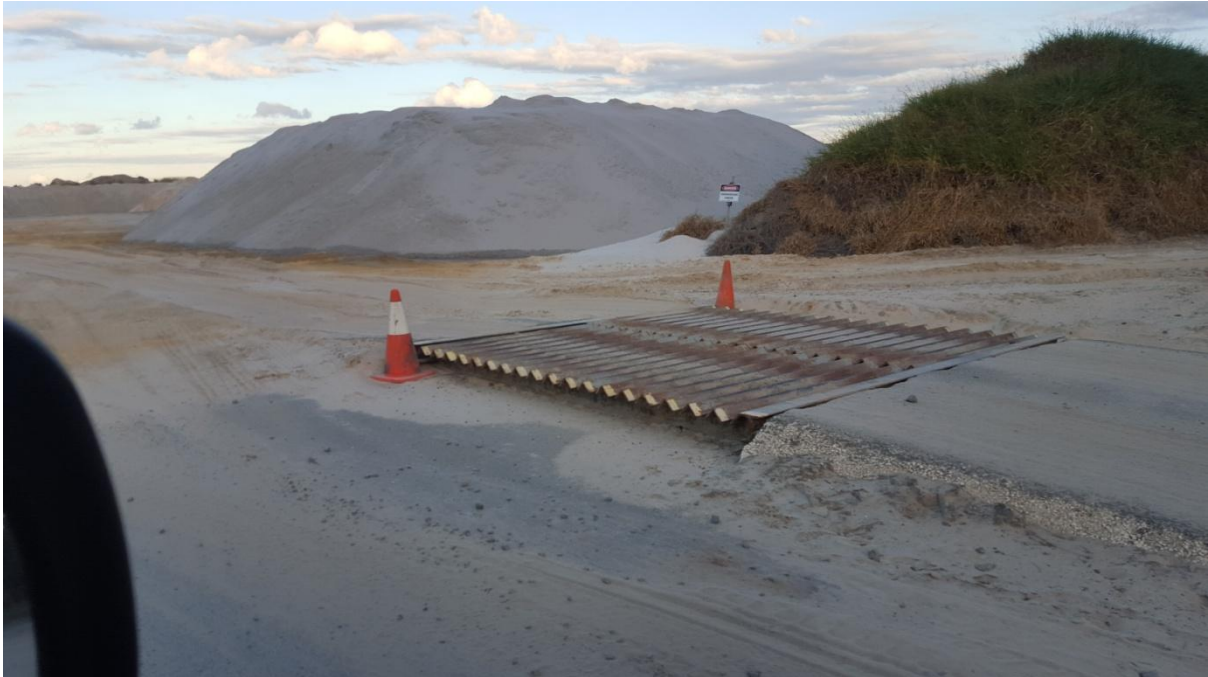
Photograph 5: Shaker grid located at entrance to operational area.
