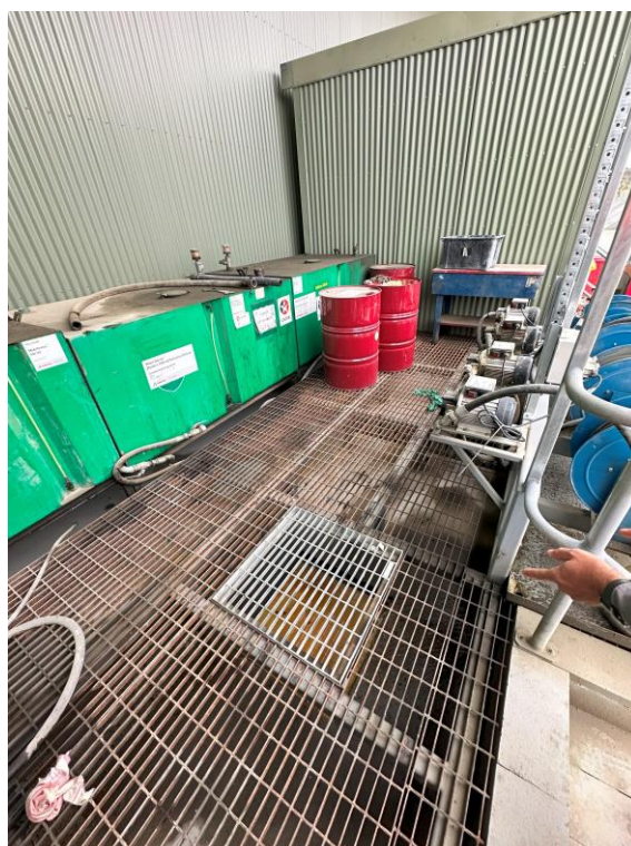
Photograph E.11 Bunded diesel storage area
