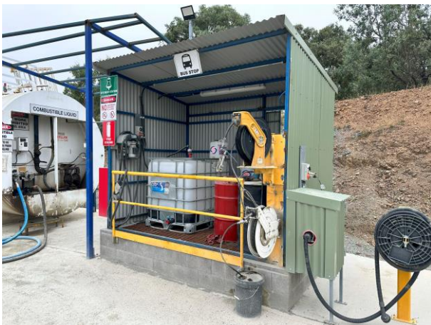
Photograph E.6 Bunded oil storage area
