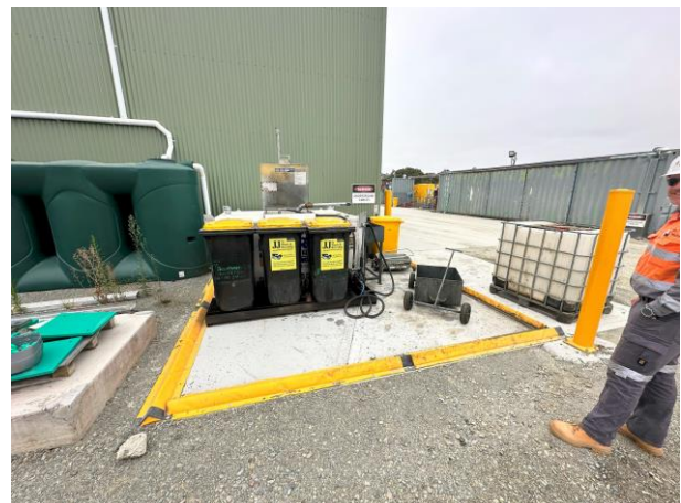
Photograph E.7 Bunded fuel and waste oil storage area
