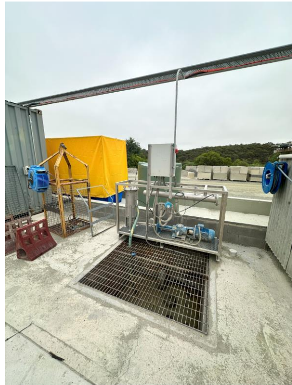
Photograph E.13 Oil separator
