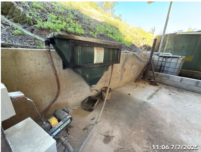
Photo 26 Oil And Water Separator
