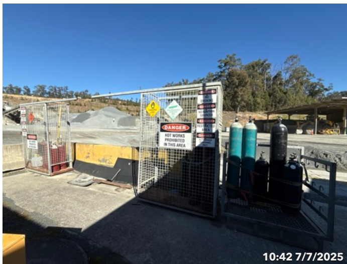
Photo 2 Gas Tanks - Chained And Secured
