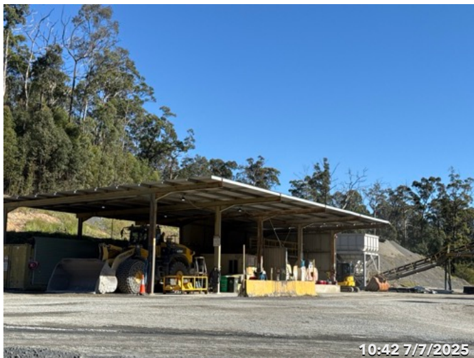
Photo 3 Bunded - Diesel And Pre-coating Tanks
