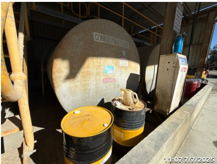
Photo 27 Bunded Diesel Tanks And Pre-coate Tank
