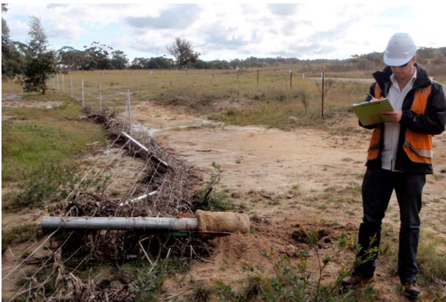
Photograph 5.5 Fencing damaged during heavy rain and surface flows (23/4/12)
