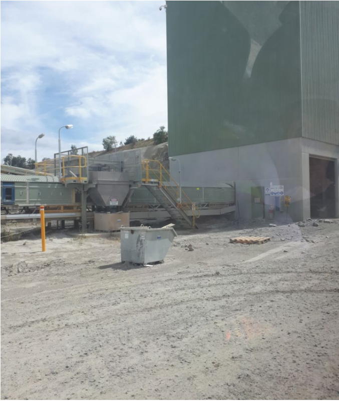
Photograph 5.8 Primary crusher area
