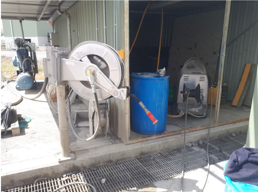
Photograph 5.6 Shed next to the main oil and chemical storage area
