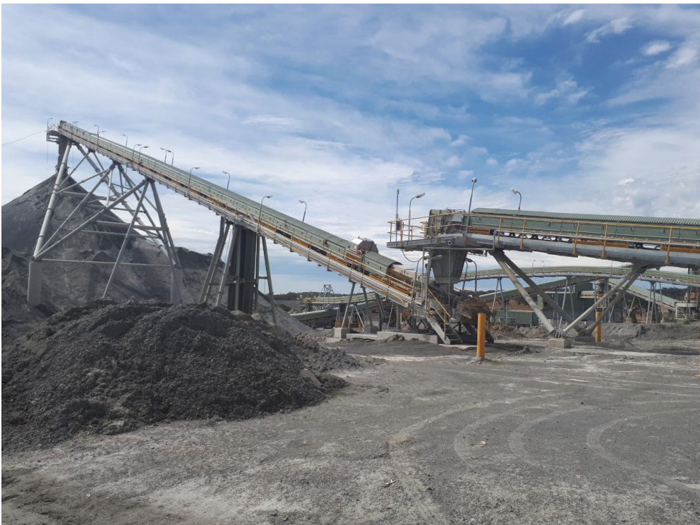
Photograph 5.2 Stockpiles and conveyor belts
