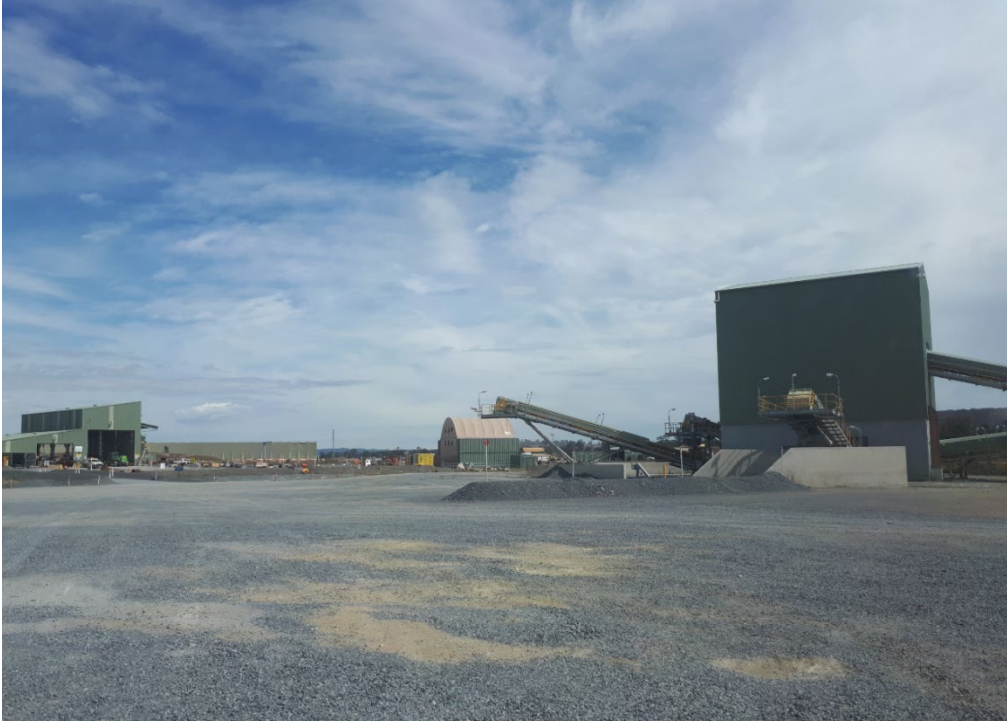
Photograph 5.1 View across the main quarry area
