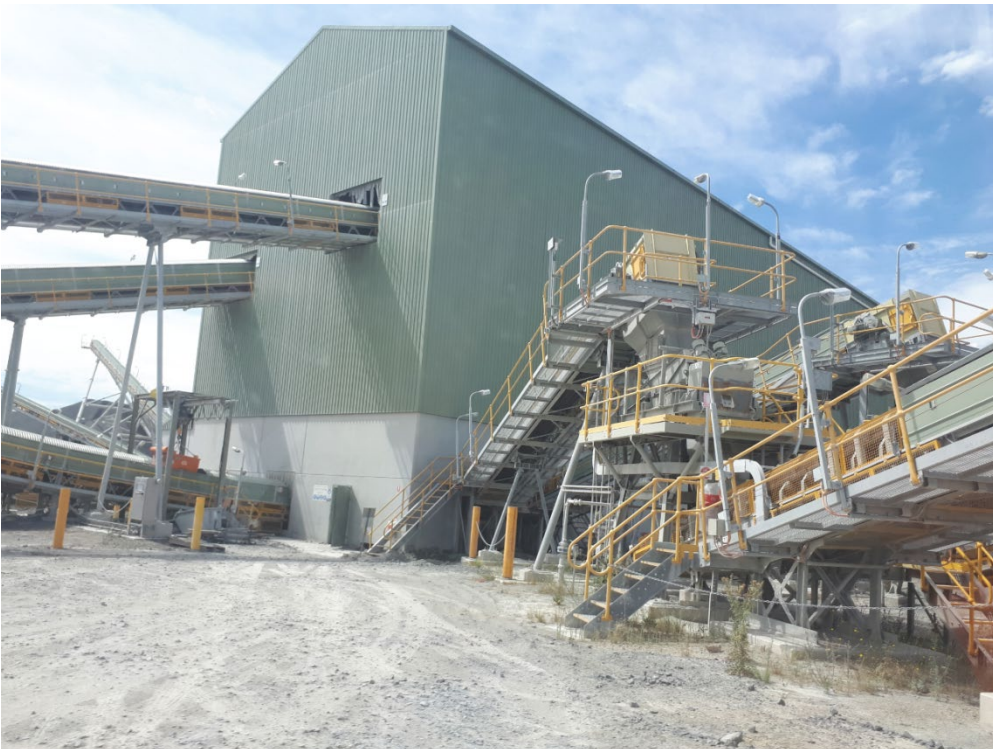
Photograph 5.4 Conveyor belts and crusher / screening building
