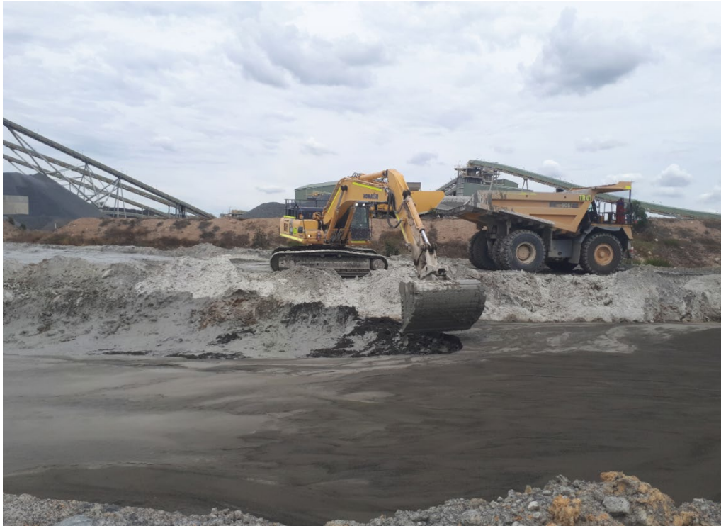
Photograph 5.9 Dam cleaning in progress
