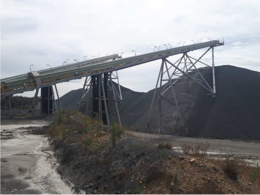
Photograph 5.3 Stockpiles and conveyor belts
