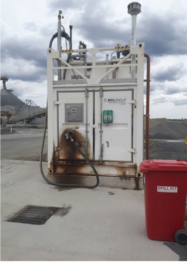
Photograph 5.11 Truck fuelling station
