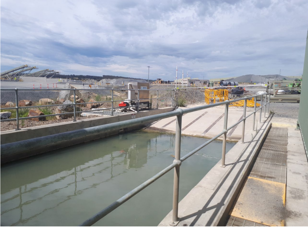
Photograph 5.7 Oil separator pit
