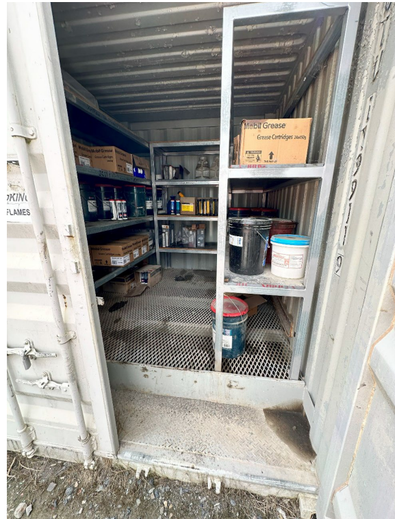
Photograph E.28 Bunded hydrocarbon storage
