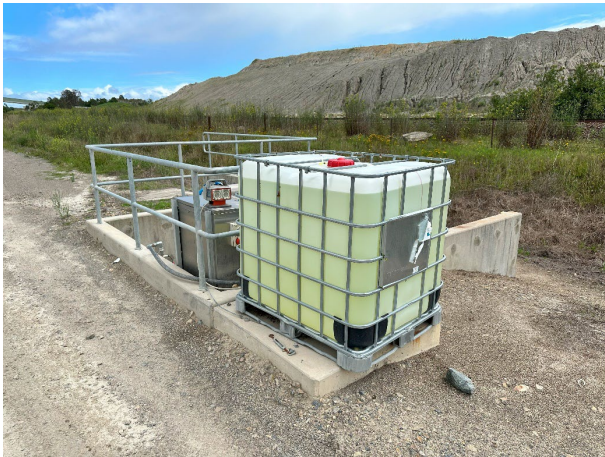
Photograph E.43 Dust suppressant and associated pump
