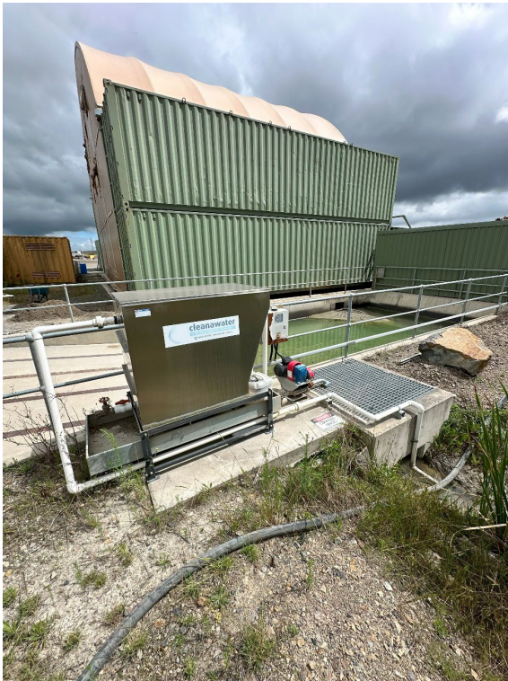
Photograph E.27 Sump oily water separator
