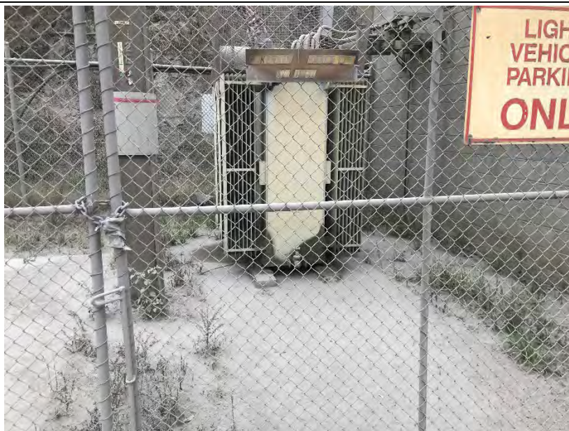
Photograph 63: Electrical transformer, shows signs of oil seepage.
