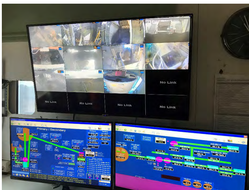
Photograph 64: Crusher control room, showing water sprays in operation. Processes are stopped if sprays are not working.
