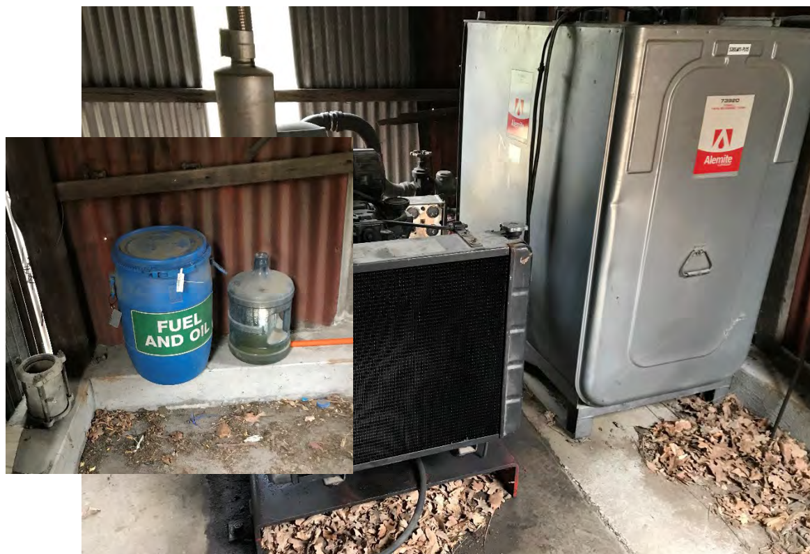
Photograph 18 – Donazzan's Dam diesel-fuelled water pump. Fuel tank is double lined. Spill kit (inset) in shed corner with inspection tag attached.
