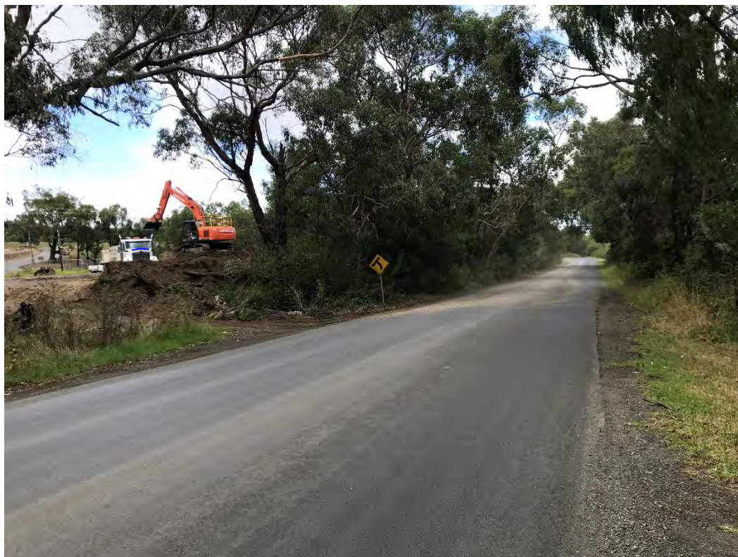
Photograph 14 – Soil being tracked from non-quarry site (left) onto lower section of Mt Shamrock Road. Quarry traffic observed to be mobilising this material causing potential local dust dis-amenity.
