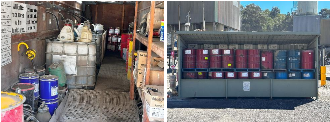
FIGURE 3: GOOD CHEMICAL, FUEL AND OIL STORAGE PRACTICES
