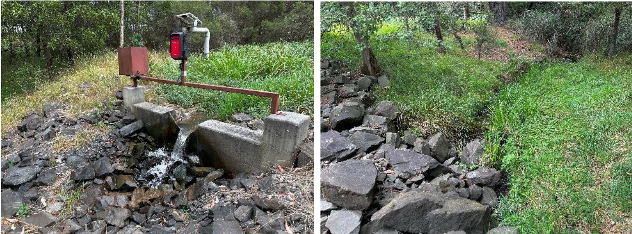
FIGURE 5: SURFACE WATER EPA LICENCED DISCHARGE POINT
