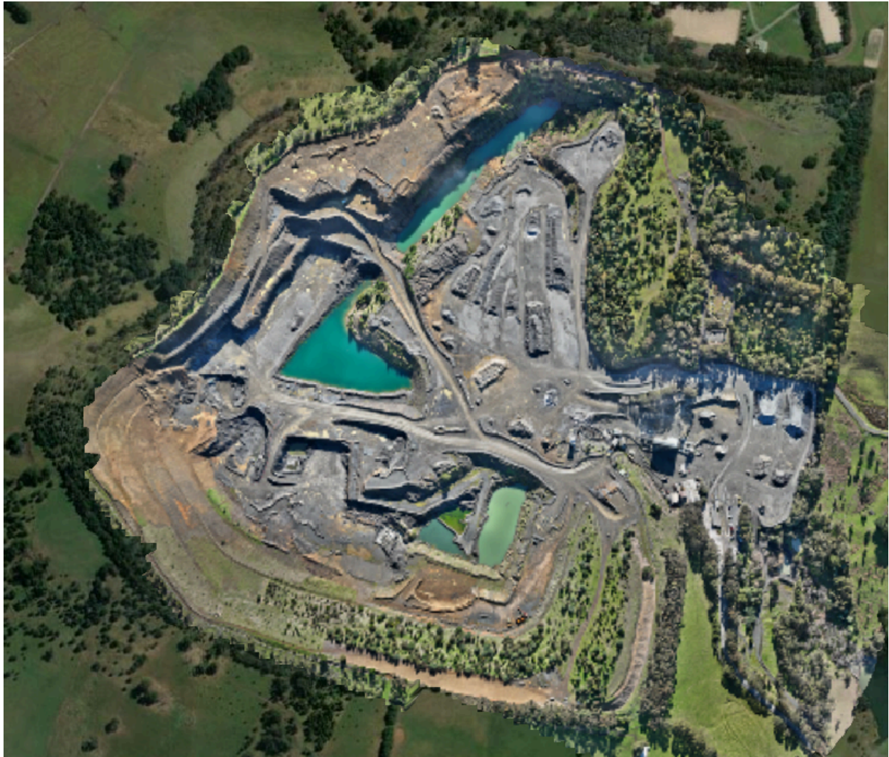
Figure 1 - Site Aerial 3rd July 2024
