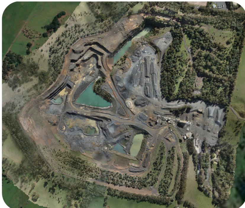
Figure 1 - Site Aerial April 2026
